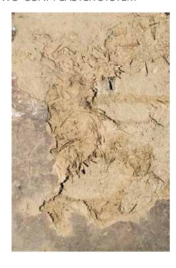
Fig. 197: The two-coat plaster support.
