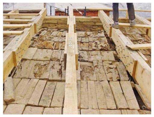
The historic ceilings and timber roof would be retained intact, conserved, consolidated and secured from the top but relieved of the unbearable weight. In addition, it would be protected by a new structural system comprising of nine beams and a layer of new ceiling planks laid on beams and new wall plates.
