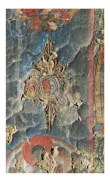
Right: Fig. 230: Losses near ground caused by water and soluble salts, apse in Lotsawa Lhakhang.
