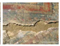
Fig. 236: Crack with old infill, Lhakhang Gongma.
