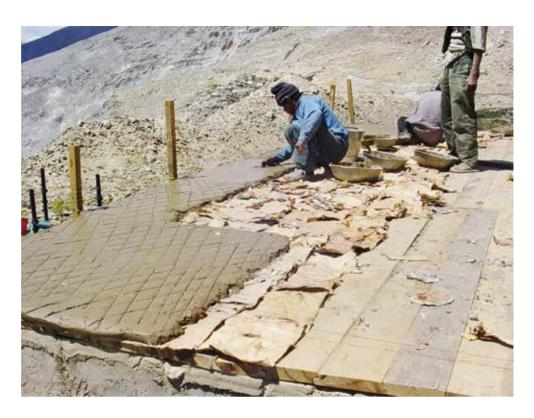
Fig. 58: Flat compacted mud roof being reconstructed at Nako.
