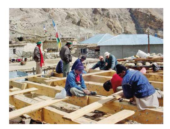
Fig. 184: New cedar beams are placed over historical roof.
