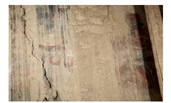
Fig. 242: Cracks and drips with clay deposits, apse in Lotsawa Lhakhang.
