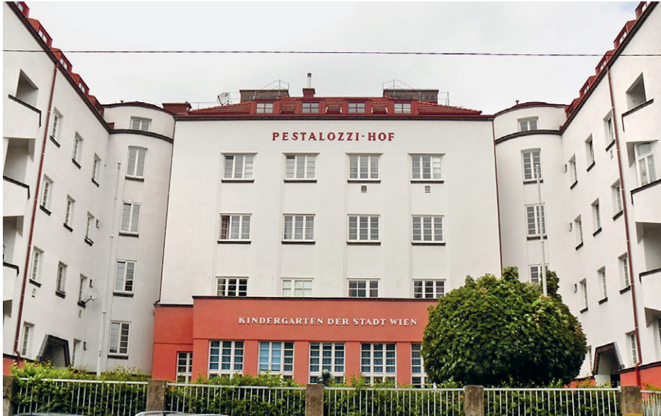
99. Ella Briggs, Pestalozzi-Hof, Wien 19, Philippovichgasse 2-4, erbaut 1925/26/Prokop
