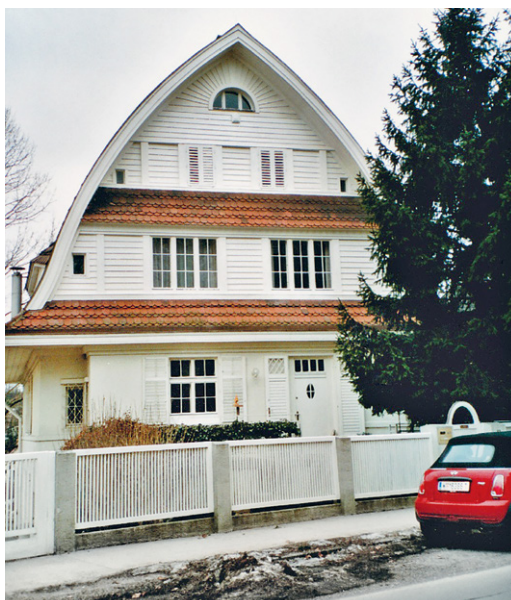
85. Karl Jaray, Villa Jaray, Wien 19, Langackerergasse 22/Prokop
