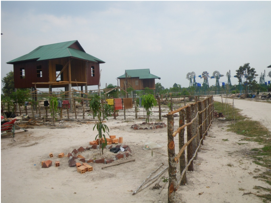
Fig. 2: Houses under construction in Run Ta-Ek (2011).
