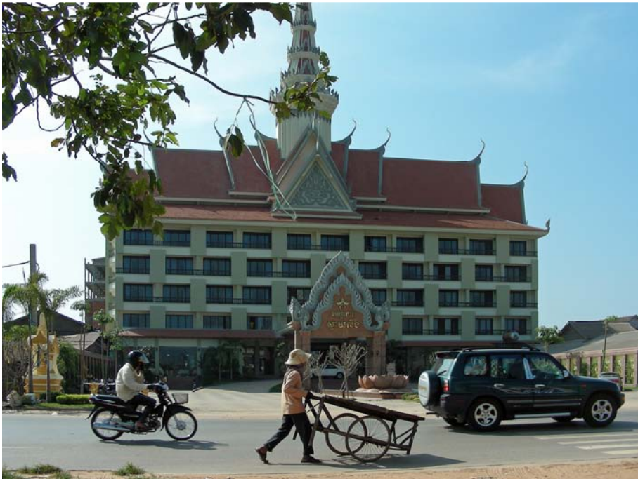
Fig. 5: New hotel with a roof in the form of a Buddhist monastery (pagoda) (2011).
