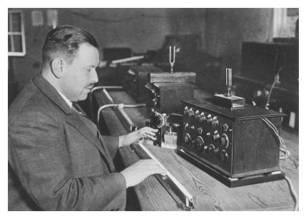
**FIGURE 18.** Friedrich Trautwein with the first model of the Trautonium, circa 1930. Source: Leo Kestenberg, ed., *Kunst und Technik* (Berlin: Wegweiser-Verlag, 1930), 452.
