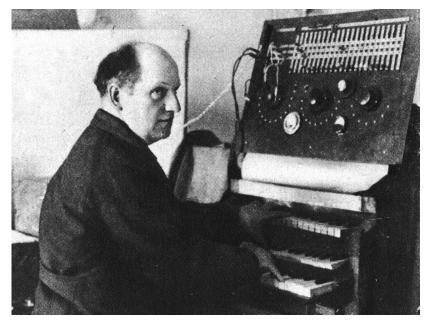
**FIGURE 13.** Jörg Mager playing the three-manual Partiturophon, circa 1930. Note how his left hand is fingering keys on both the upper and the middle manual: this technique was required for polyphonic playing, as each manual could sound only one tone at a time. Source: Andy Mackay, *Electronic Music* (Minneapolis: Control Data Publishing, 1981), 19.
