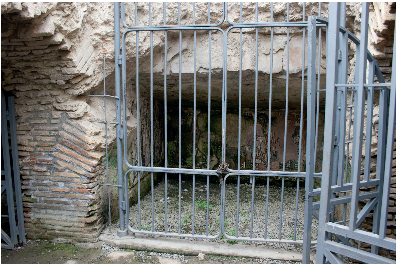
Fig. 4: Western alcove, view from east (Photo: G. Fingarova).
