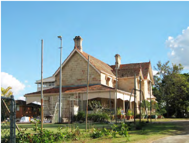
Illustration 11. Bulimba homestead, now located in the Brisbane suburb, Bulimba.
