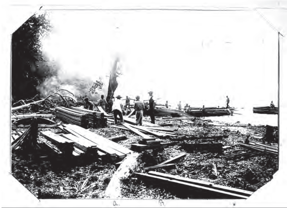
Figure 29. 'Unloading timber for Govt. Residence and Lock up at Tulagi. Photographed by Mr Lucas SS 'Titus'. a. Resident Commissioner. b. The Carpenter'.
