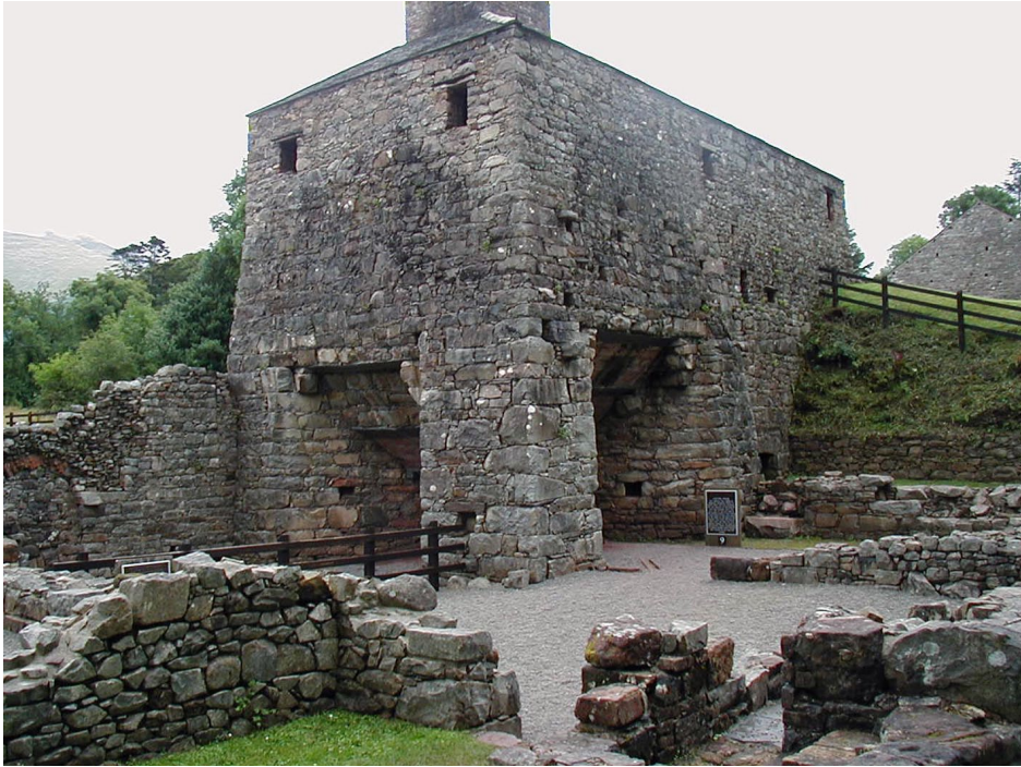
Figure 1.2: The Lorn Furnace at Bonawe on the banks of Loch Etive.
