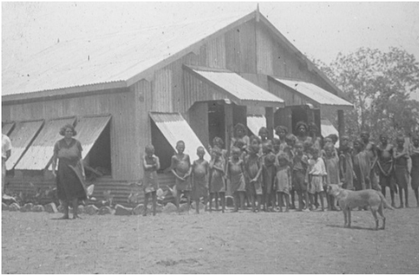
Figure 9.2: The new School at Roper Mission 1937.
