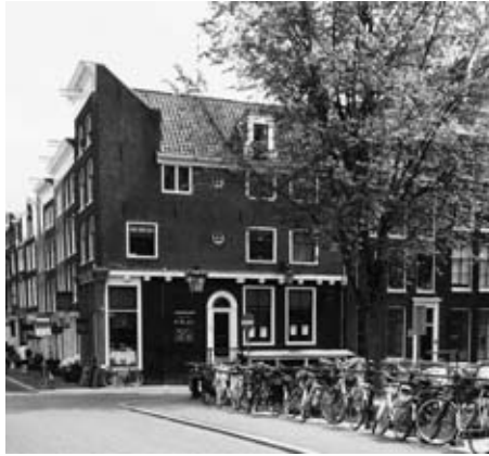
12.5. Amsterdam, Keizersgracht at the corner of the Herenstraat. The house was rebuilt in 1967 incorporating its ruinous bottom half. With the aid of the Grachtenboek the upper half was reconstructed, adding an extra row of windows on the Herenstraat side. (Photo: F. Schmidt).
