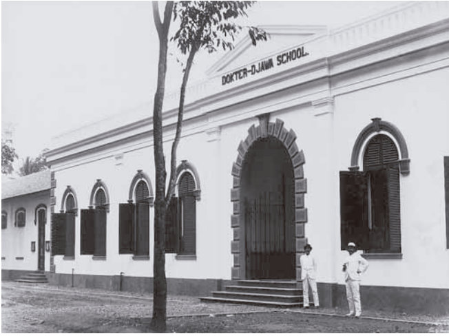
The new school building (photo collection KITLV 35810)
