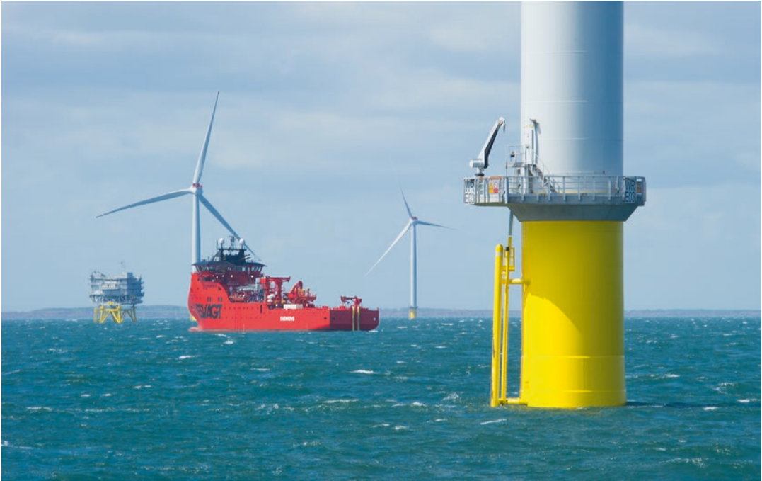
Fig. 26.2 The Westernmost Rough offshore wind farm under construction, located 8 km offshore of the Yorkshire coast near the Humber estuary, giving some idea of the infrastructure involved in wind farm installations. The total array covers an area of 32 km 2 with 35 turbines, three of which are visible in this photograph, connected by 53 km of submarine cables, and an offshore electricity substation, visible on the far left. The red ship is a specialist vessel for servicing the turbines. © Historic England Archive, Alun Bull
