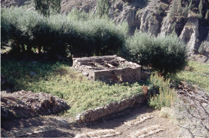
FIGURE 6.6 Dilapidated shrine. Lha Lama Temple (Tib. lha bla ma lha khang ). Johling, Lahul. Dated to the time of Rinchen Zangpo. VERENA WIDORN, 2002, WHAV
