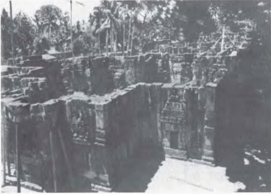
Photo 17. Mock-up or trial reconstruction of a horizontal section of the wall of the Śiva temple (OD 13297, reproduced from Djāvā 20 (1940))
