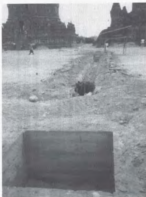
Photo 3. Recent drainage measures in the western part of the central temple area (photograph by Pia Hoekstra)
