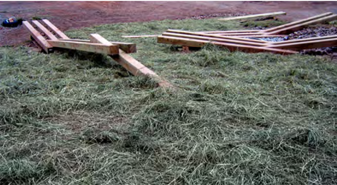
Image 3: Cheticamp, Nova Scotia Construction, NAR 2006
