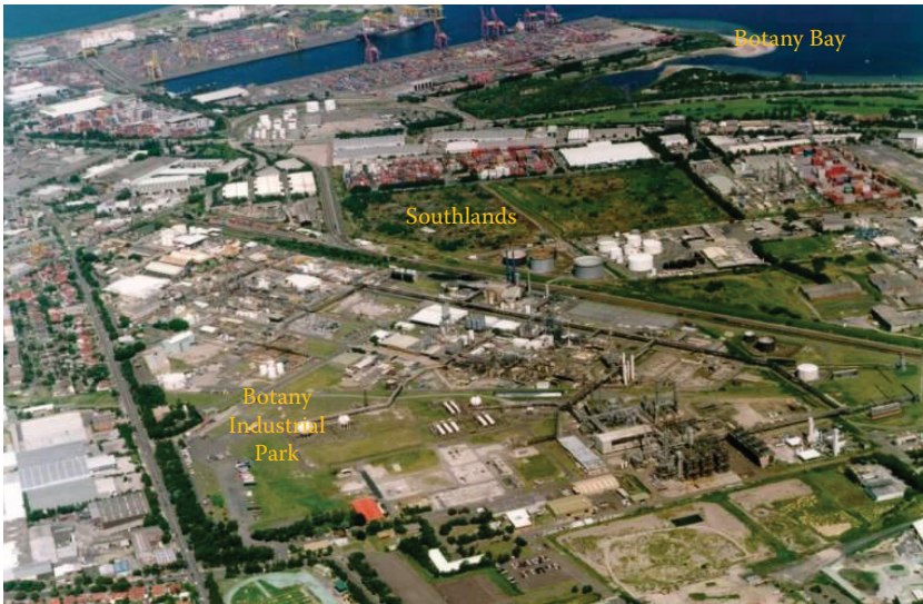
FIGURE 12.2 BIP and surrounds. (From Orica Ltd.)
