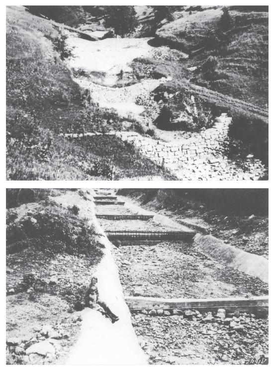
*Figure 4.9* Examples of elaborate drop structures to control hillside gullies creating rock fans on transportation routes. Top: Near Genoa, WI, to protect railroad, 6/27/30. Bottom: Between Wabasha and Lake City, MN, 1932. (Photos credit: C.G. Bates.)
