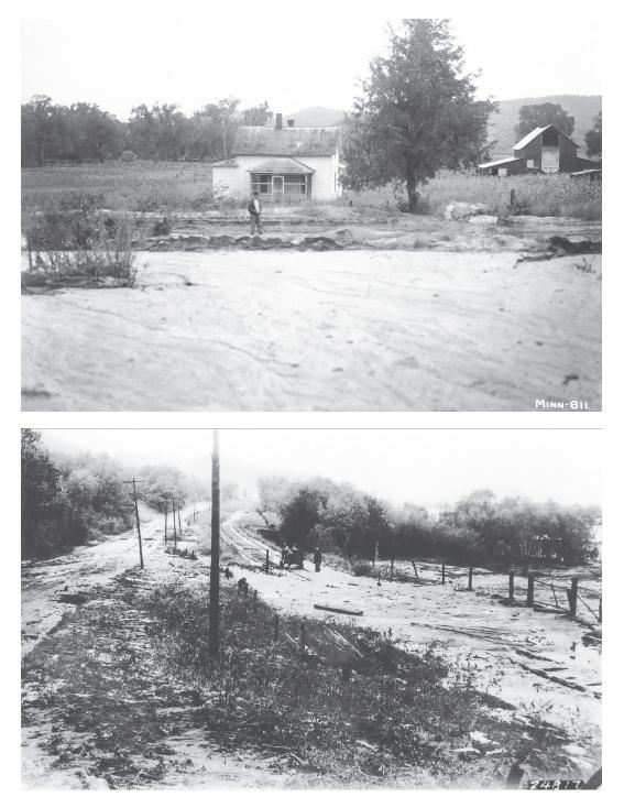
*Figure* 4.7 Examples of gully fans covering roads and railroads. Top: Sand fan over MN highway 74, 2 mi (3 km) west of Weaver, 9/7/38, looking south. (Photo credit: Vince McKelvey). Farm in background was already abandoned. Bottom: sand fan over railroad, location unknown. (Photo credit: C.G.Bates, 8/2/30.)
