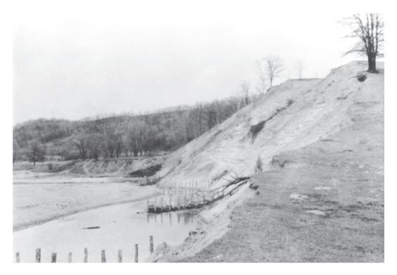
*Figure 2.16* CCC project to stabilize high Pleistocene terrace undercut by stream. Exact location unknown but probably Trempealeau Co., WI, late 1930s. SCS Photo.
