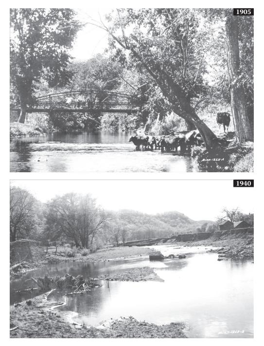
*Figure 5.5* Fairwater, bridge crossing visible in 5.1 and 5.2 looking upstream. c. 1905: the structure is probably slightly later than the one visible in 5.1 and 5.2 but is at the same crossing. Note stability of stream and banks. 1940: stream widened by about three times here so that right pier is near the center of the widened stream. The left pier is still visible (2006) in the village, but the recovering (narrowing) stream has buried the right pier in the new bank.
