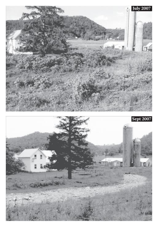
*Figure 8.7* Flume formed from rock fan to protect farm, similar to that at Zink farm (see Figure 8.6), photo made from County P looking north, Timber Coulee, NW1/4, Sec 8, T14N, R4W, Vernon Co. P = 7–8 in. (20 cm). Top: July 2007, dormant flume. Bottom: September 2007. Note "gravel road" appearance. (Photo credit: Edyta Zygmunt.)
