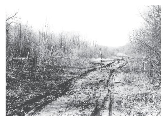
*Figure 7.22* Minnesota State Aid Highway 9 on the south side of the Whitewater River, 11/6/37. Bridge in right foreground was covered by 18 in. (45 cm) of sediment by June 1938. This road, the lifeline for people on the south side of the river, was becoming impassable by the late 1930s. By 1989, it was underwater, impassable even on foot. (Photo credit Soil Conservation Service [SCS].)
