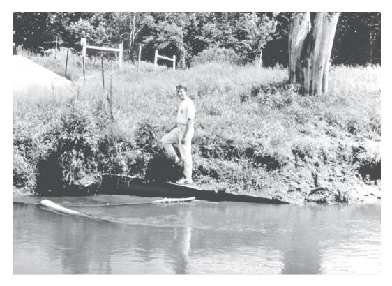
*Figure* 7.23 The south abutment of an old Dodson Hollow Road bridge over Coon Creek (SE1/4, Sec 22, T14N, R6W, Vernon, Co., WI). This bridge was replaced in 1926 as the creek rapidly aggraded, and the abutment was later buried in the floodplain. When built, probably in the early 1900s, this abutment was at least 10 ft (3 m) above the water. A small lateral shift by the stream in 1993 exposed the old abutment. The newest bridge (c. 1990) is seen to the far left.
