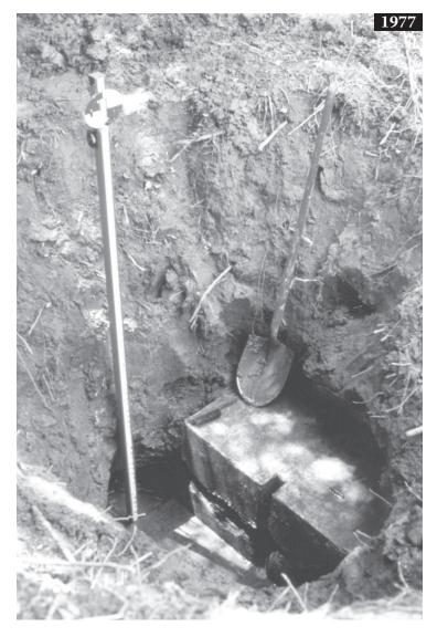
*Figure 7.5 (Continued)* 1977. Rectangular pier to hold flashboards (seen in the 1946 photo), excavated 1977. An elevation placed on the dam in 1932 tied into earlier surveys by the WI Dam Commission and allowed reconstruction of village elevations back to 1914 (Figure 7.2).
