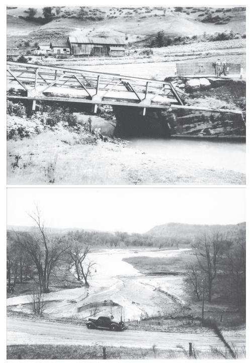
*Figure 5.10* Bridges over tributaries destroyed by flooding and sediment. Top: Undermined bridge in the Coon Creek basin, exact location unknown, 1938 (from McKelvey, V.E. 1939. Stream and valley sedimentation in the Coon Creek drainage basin, Wisconsin: M.A. thesis, University of Wisconsin-Madison). Bottom: Abutment of destroyed bridge over Trout Brook near Dumfries, MN. Zumbro River Valley, 1939 (Sec 10, T110N, R11W, Wabasha County) (SCS Photos).
