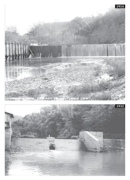
*Figure 7.5* The main dam at Chaseburg looking upstream; refer to Figure 7.2. Top: wooden dam in 1914 at head of shoals. The race on the left extends 140 ft (44 m) to the mill, which originally gave 3 ft (1 m) more head or fall. This much fall meant that the dam was built on bedrock and that the bedrock extended at least to the mill. Bottom: Concrete dam built downstream at mill in 1932. Note sluice gate (center). (Continued)
