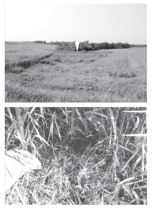
*Figure 8.4* A sediment trap after the 2007 storm. Top: A "dry" floodwater retarding dam (arrow) controlling about 8–10 acres (3–4 ha) of mostly no-till crops, 5 mi (8 km) north of Altura, MN, on Beaver-Altura Road looking west. P = 10 in. (25 cm). Corn is to the left and soybeans are to the right. Bottom: Bottom of dry pond. Note lack of any sediment accumulation. NW1/4, Sec. 19, T18N, R9W, Winona County, MN. Photos made Sept. 2–9, 2007.
