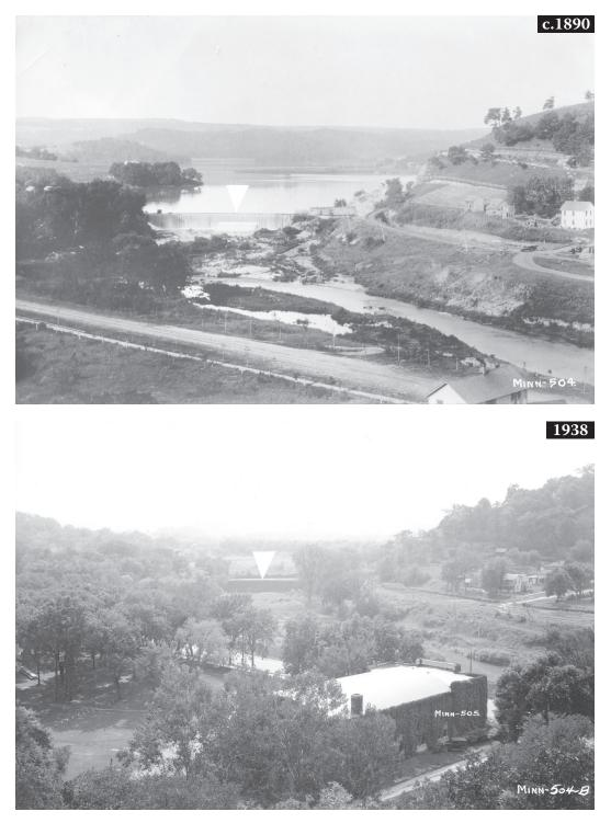
*Figure 5.13* Lanesboro Lake, Lanesboro, MN, on the upper Root River. C. 1890: large expanse of water. 1938: completely filled with sediment. Arrow marks top of dam in both photos. (Photo credit Soil Conservation Service [SCS].)
