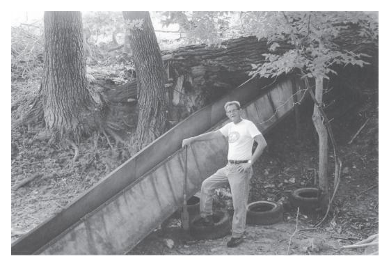
*Figure 3.5* Early private erosion control. Sheet metal flume used to convey water around the head of gullies, Proksch Coulee gully, Vernon Co., WI (see Chapter 4). (Photo credit: Nadine Kleinhenz.)
