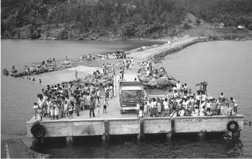
FIGURE 10.3. Modern Ro-Ro berth at Kadavu Island, Fiji, and adjacent platform for landing craft and barges. (Photograph by the author, 1986)
