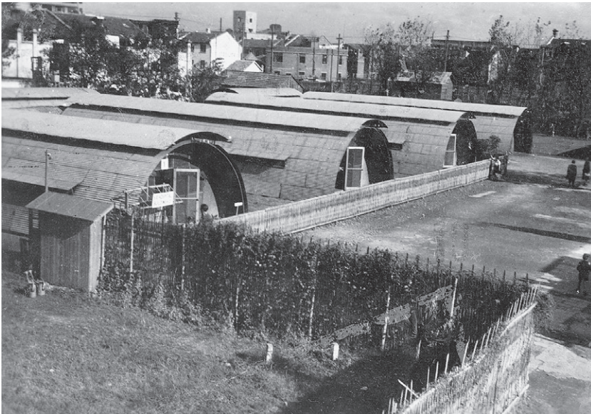
Fig. 12: Seward Road camp opened in 1942. It could shelter 1000 refugees and operated the central kitchen, which served daily meals to some 8000 refugees (c. 1942–1945).
