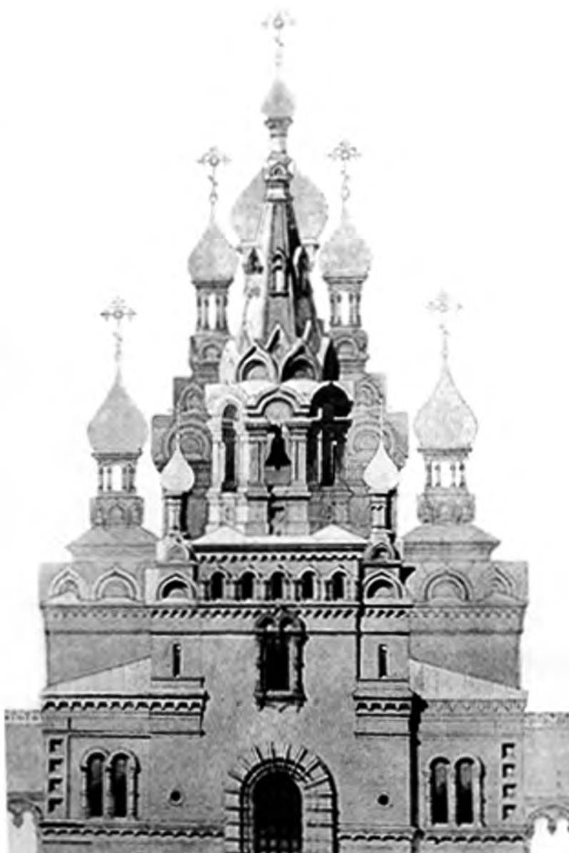
Figure 7—Alexander Gogen—Orthodox Church, Port Arthur. Stroitel' , 1902
