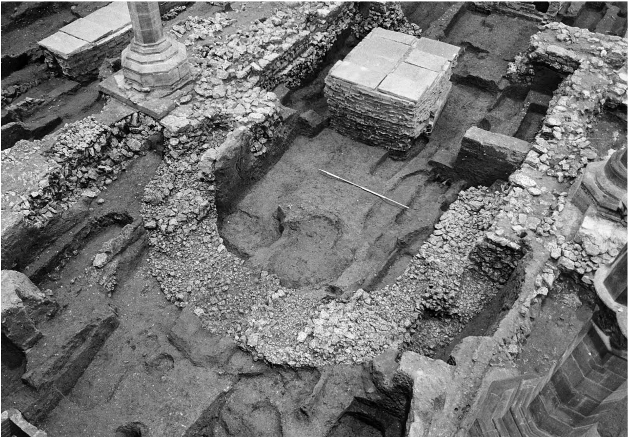
Fig. 392: Foundations of the chancel and apsidal sanctuary of the Period 3 church. View south-west. Scale of 2 m. Photo: Warwick Rodwell
