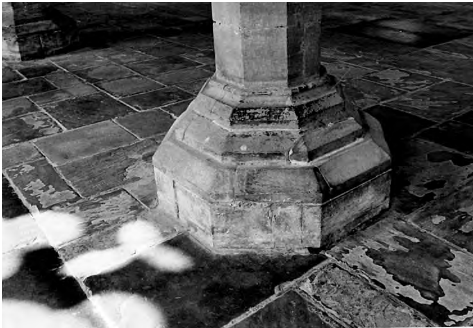
Fig. 496: South arcade. Base of pier 2/3, from the south-east. Photo: Warwick Rodwell
