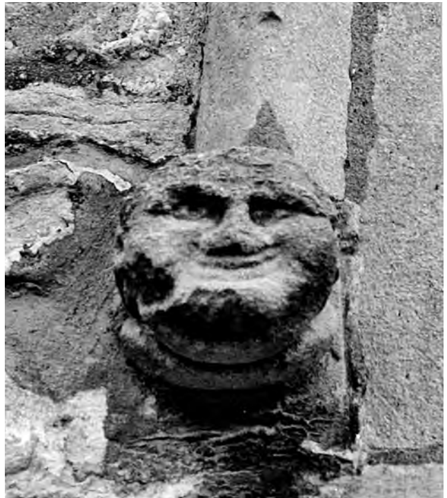
Fig. 532: North aisle window, bay 4. West label-stop, no. 49. Photo: Warwick Rodwell
