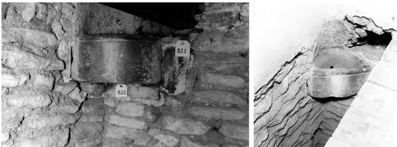
Fig. 580: Tower. Two views of the quadrant-shaped limestone bowl, probably originally a stoup, reset in the south-west corner of the ringing-chamber for use as a bellringers' urinal. Photos: Warwick Rodwell
