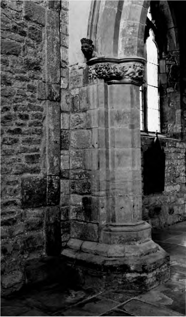
Fig. 492: North arcade. West respond, from the south-east, showing also the abutment of the arcade to the long-and-short quoin of the late Saxon tower. Photo: Warwick Rodwell
