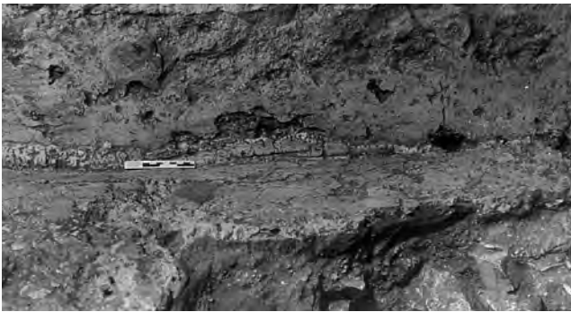
Fig. 423: Tower: interior. Lime concrete floor of Period 3 abutting the west wall. Note how the new floor has been joined into the damaged earlier wallplaster, just above the scale of 8 cm. Photo: Warwick Rodwell
