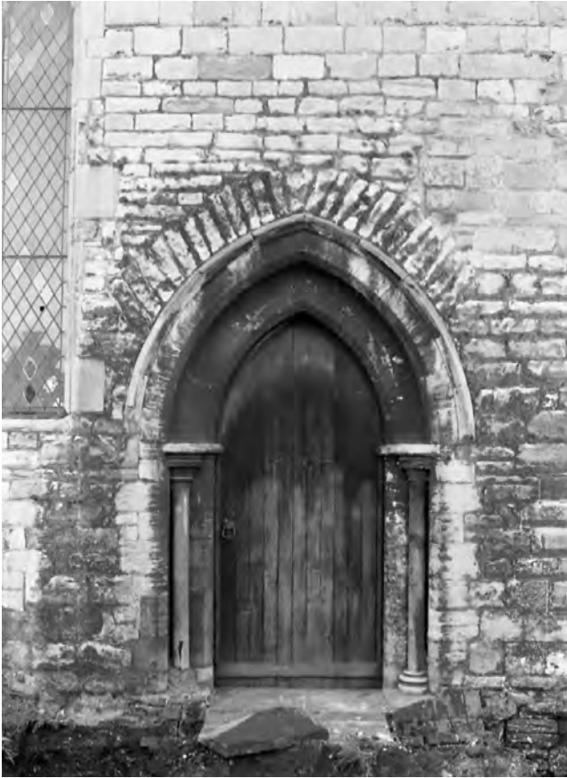
Fig. 81: St Mary's: north doorway, 1980. Photo: Warwick Rodwell
