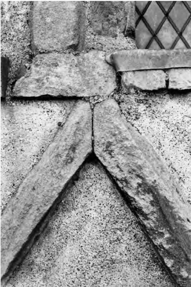
Fig. 365: St Peter, Barton-upon-Humber. Tower: Stage 1B. Detail of stone jointing from the triangular-headed arcading on the north elevation, showing a carpenter's mitre. Photo: Warwick Rodwell
