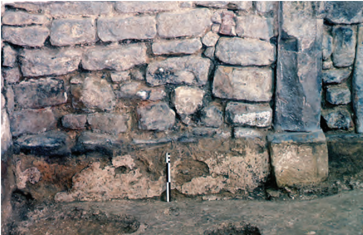
Plate 29: Tower. Surviving band of primary plaster at the base of the east wall, abutting the base for the pilaster-strip flanking the chancel arch. Note how the lower end of the pilaster is spalled as a result of fire. View east. Scale of 25 cm. Photo: Warwick Rodwell
