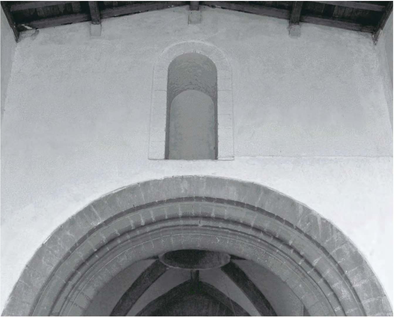
Fig. 388: St Kyneburgha, Castor (Cambs.) . High-level doorway at the east end of the nave. Photo: Warwick Rodwell
