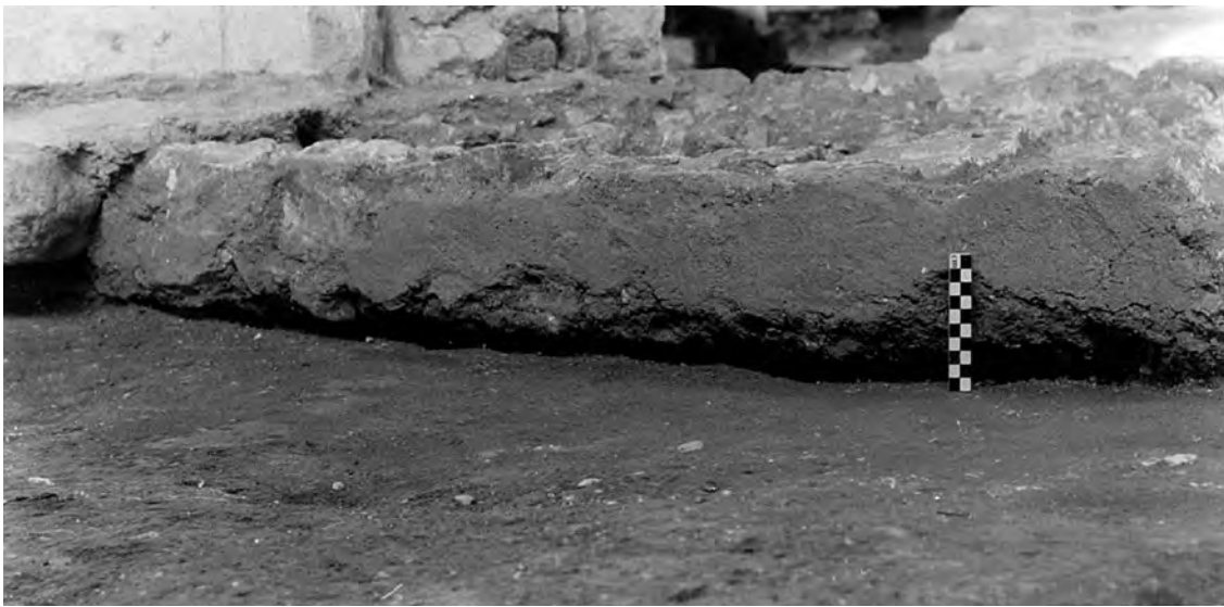
Fig. 397: Saxo-Norman nave. Primary rendering surviving at the base of the north wall. Scale of 10 cm. Photo: Warwick Rodwell
