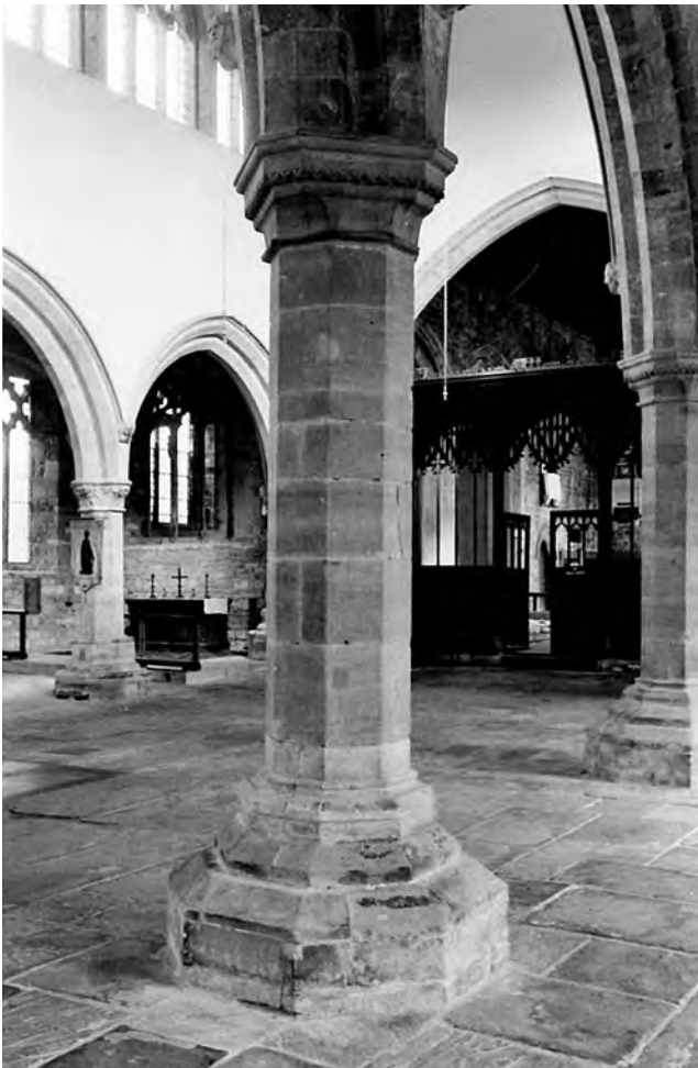
Fig. 494: South arcade. Pier 3/4 from the south-west, 2005. Photo: Warwick Rodwell
