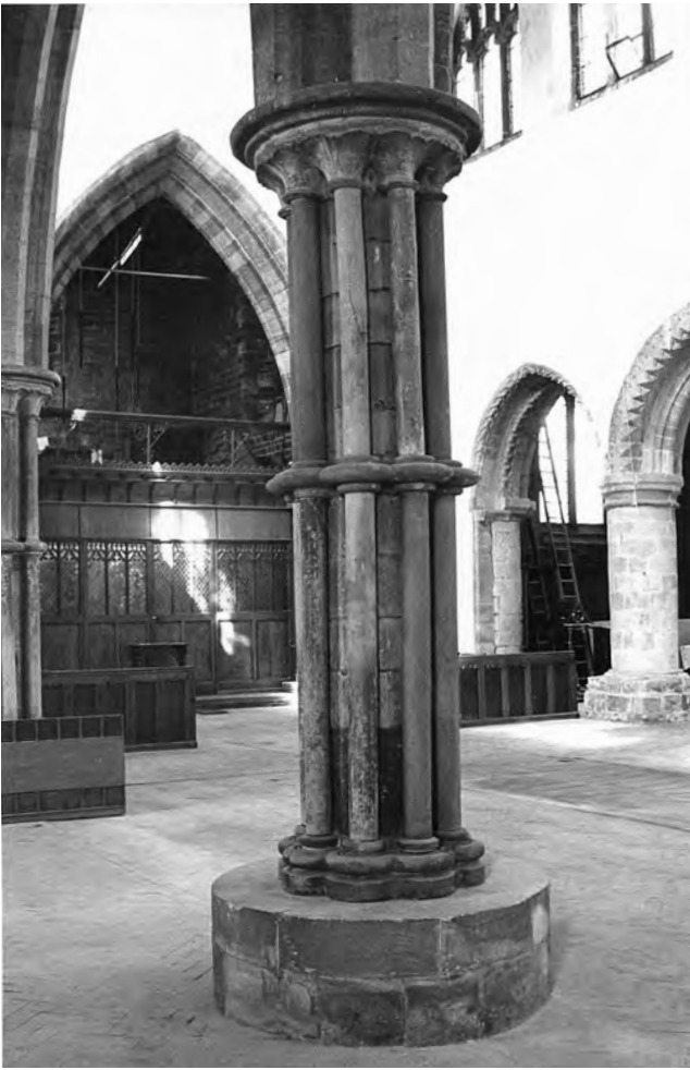
Fig. 68: St Mary's: south nave arcade, 1984. Clustered pier with basal seat in bay 2/3; view from the south-east. This pier was rebuilt in 1892. Photo: Geoffrey Bryant
