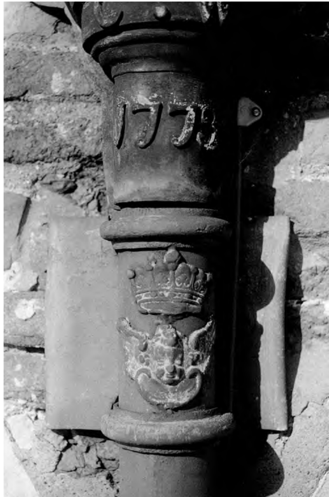
Fig. 584: South clerestory, central rainwater pipe. Detail of the dated hopper-head and cast lead plaques on the uppermost collar of the downpipe. Photo: Warwick Rodwell
