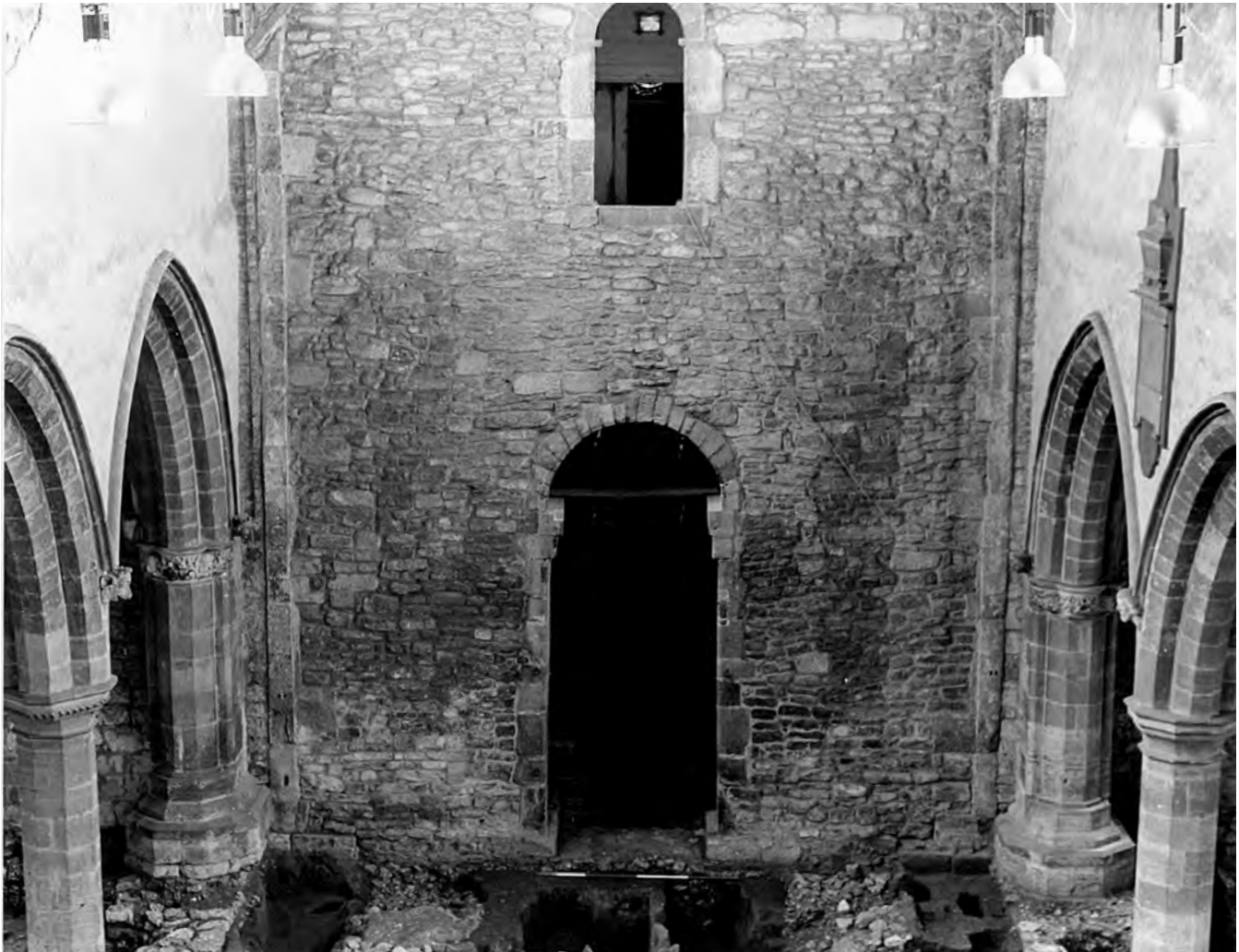
Fig. 347: Tower: east face, showing bonding scars (patched with darker coloured rubble), where the Anglo-Saxon chancel walls were formerly attached. Scale of 2 m. Photo: Warwick Rodwell
