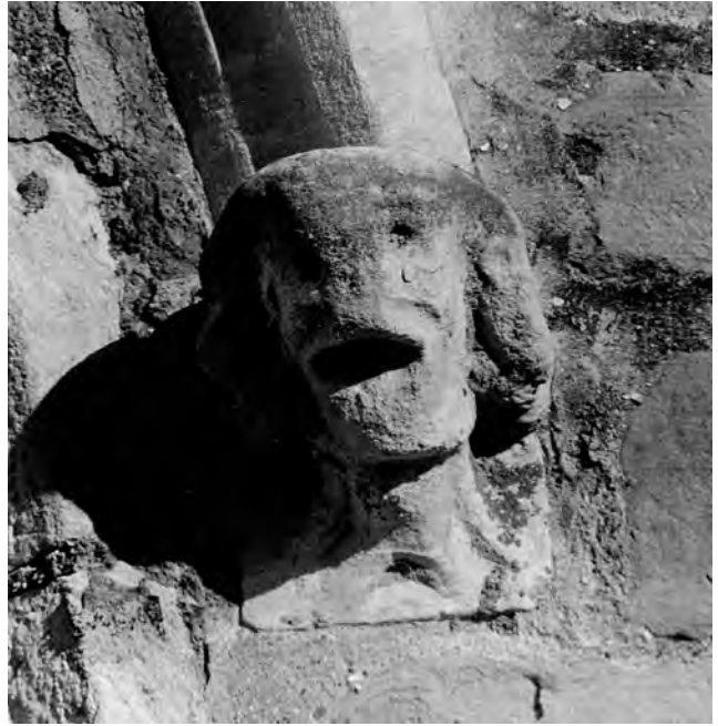
Fig. 530: South aisle window, bay 4. East label-stop, no. 42. Photo: Warwick Rodwell
