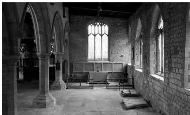
Fig. 629: South aisle, looking east, 2005. Photo: Warwick Rodwell
