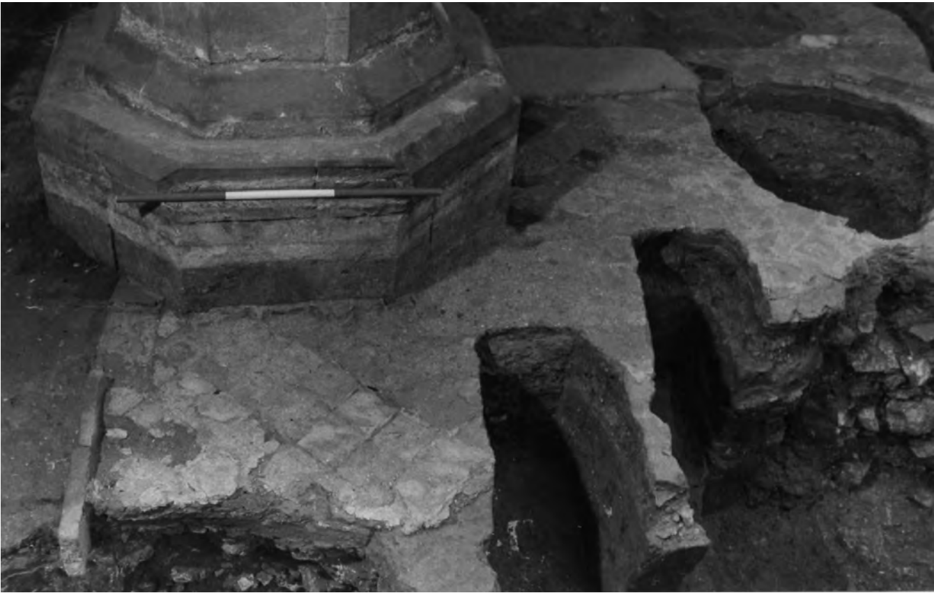
Fig. 833: Mortar bedding for a tile floor (Area E, F12) in bay 5 of the nave, abutting pier 4/5 of the north arcade. Note the brick-on-edge (left) defining the limit of the paving. View east. Scale of 75 cm. Photo: Warwick Rodwell
