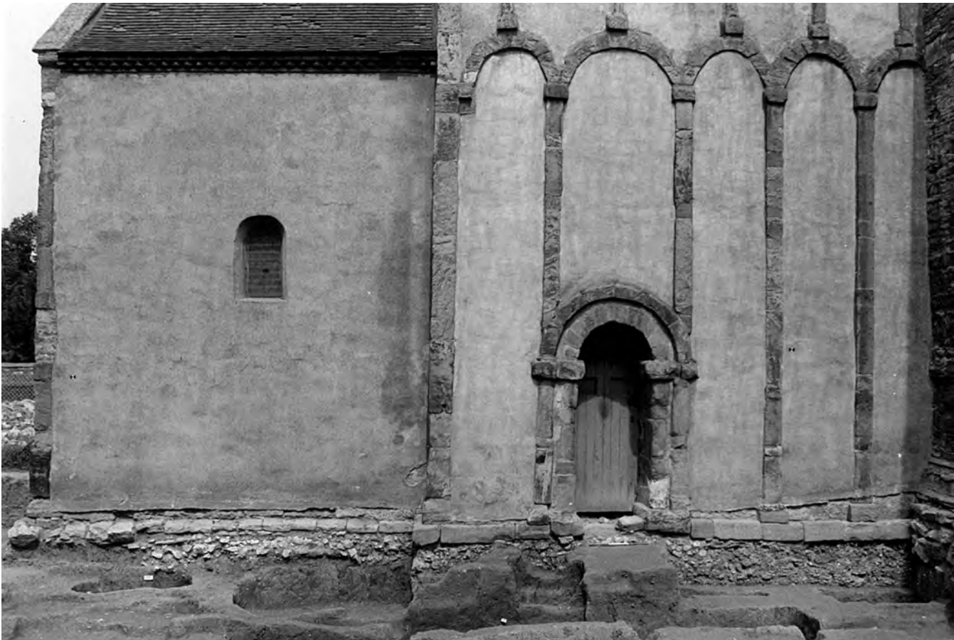
Fig. 260: Tower (Stage 1A) and annexe from the south, after excavation, 1981. Photo: Warwick Rodwell
