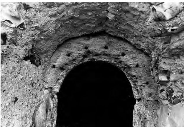
Fig. 332: St Botolph, Hadstock (Essex) . Semicircular head of a jointed window frame in the nave, showing the arc of small holes used to anchor the basketwork hood which served as a former for the arch of flint rubble. Note the preserved wattle impressions in the soffit. Photo: Warwick Rodwell
