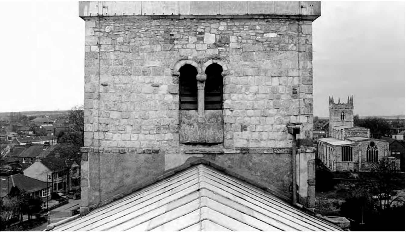
Fig. 408: Tower: Stage 3, east face. Saxo-Norman belfry in 2000, with St Mary's church beyond. Photo: Warwick Rodwell
