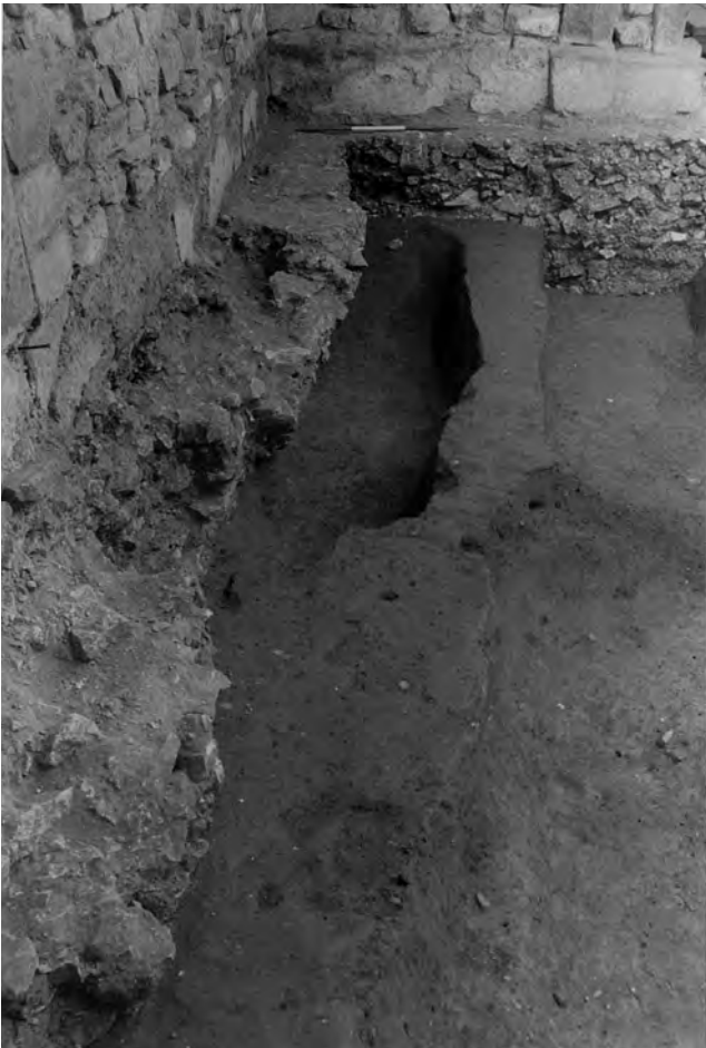
Fig. 304: Tower: interior. Irregular outline of the foundation on the north side (left), resulting from the slumping of the unstable fillings of exhumed graves. View east. Scale of 75 cm. Photo: Warwick Rodwell
