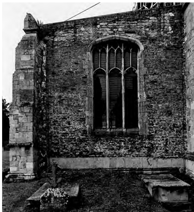
Fig. 561: South aisle. East wall unrestored, 1999. Photo: Warwick Rodwell
