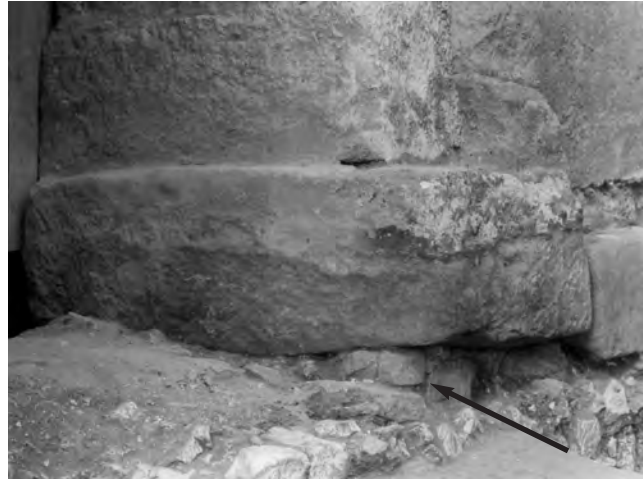
Fig. 306: Tower: south doorway, eastern jamb. Detail of the gritstone base, with masons' waste used as packing material for levelling the block. Photo: Warwick Rodwell
