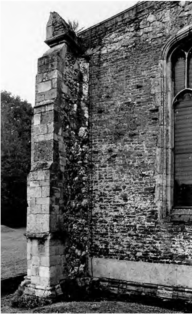
Fig. 562: South aisle. Detail of the south-east clasp buttress, showing how the Tudor east wall was set further west than its predecessor, leaving a rubble scar on the side of the buttress. Photo: Warwick Rodwell
