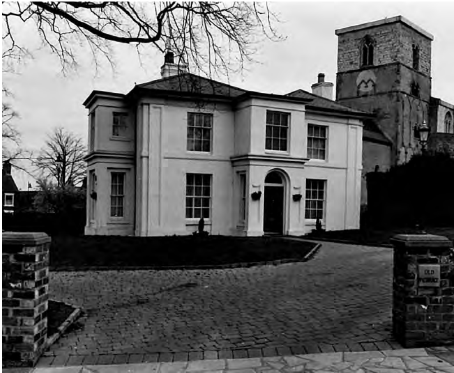
Fig. 691: Barton (old) vicarage, 2000. South side, with entrance porch of c. 1850. Photo: Warwick Rodwell
