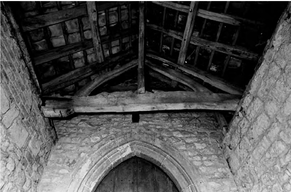
Fig. 554: North porch roof. View of the underside, 2000. Photo: Warwick Rodwell
