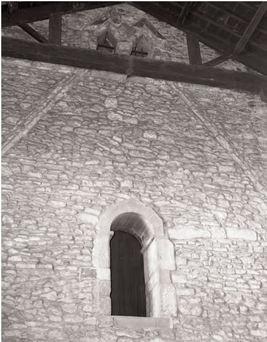
Fig. 289: Tower: Stage 1B. High-level doorway in the east wall (east face), 1972. The voussoirs and impost of the arch date from 1858. Photo: English Heritage, NMR
