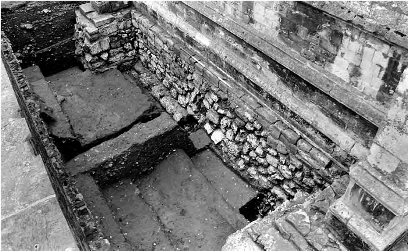
Fig. 445: Chancel, east wall: foundations and construction trench. Note the large projecting blocks in the base of the trench, representing a pre-fourteenth-century phase in the southern half of the wall (left of centre). View south-west. Scale of 2 m. Photo: Warwick Rodwell
