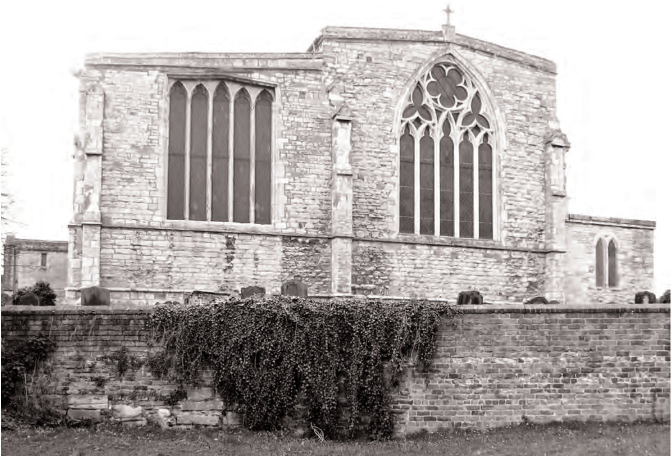
Fig. 53: St Mary's: east elevation of the chancel, south aisle and vestry, 2005. Photo: Warwick Rodwell
