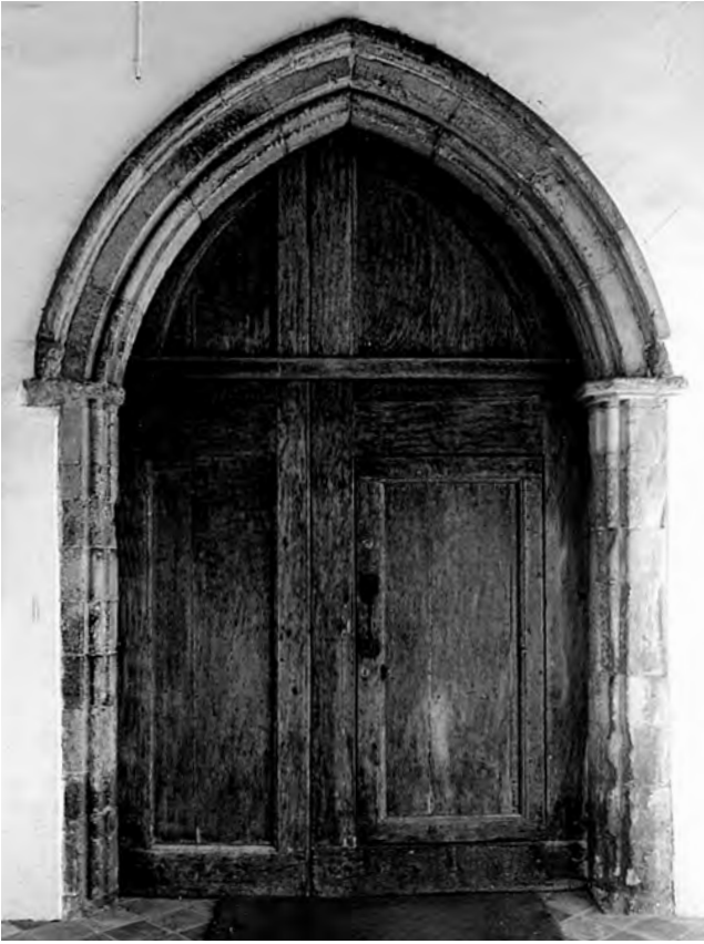
Fig. 83: St Mary's: south doorway. Photo: Warwick Rodwell
