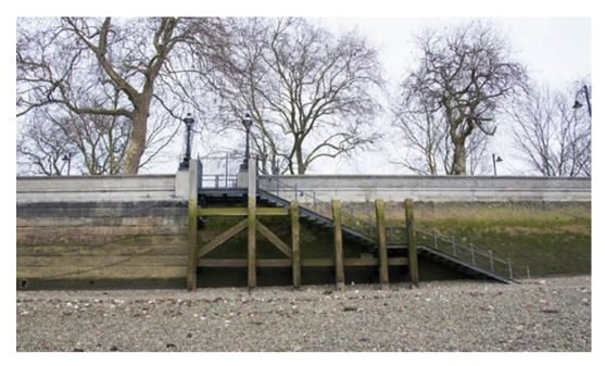
Figure 3. Royal Hospital Stairs, Chelsea. The 1850s embankment is on the right of the river stairs, and is brick built. The 1870s embankment is on the left of the river stairs and is finished with faced granite blocks (Author and Clare Dowling 2016).
