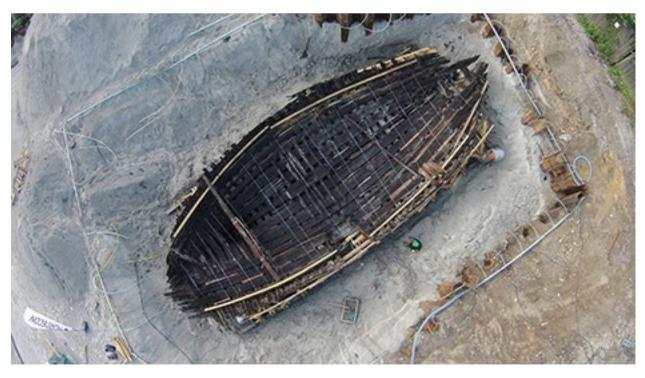
Figure 5. View of the pit of the wreck Peeter. In addition to the sheet pile wall, a well-point dewatering system was installed to enable archaeological excavations below sea level (Maili Roio).
