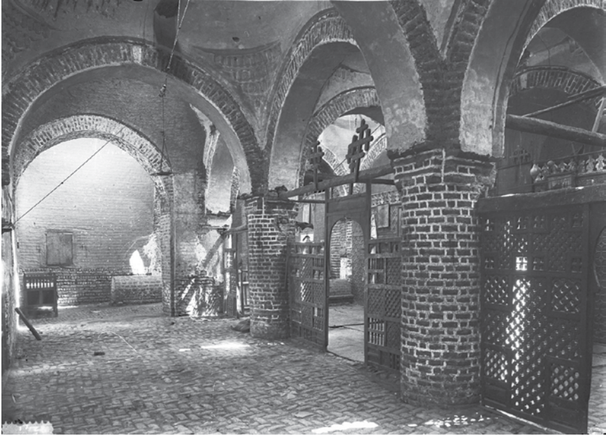
FIGURE A1.3 Interior of Coptic church (NED-B-8241)
