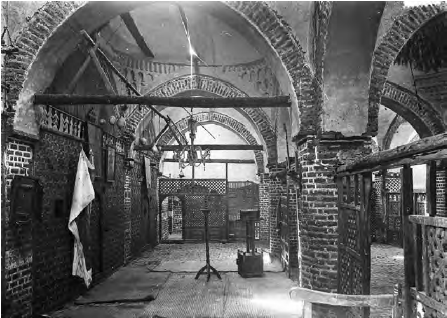
FIGURE A1.2 Interior of Coptic church (NED-B-8242)
