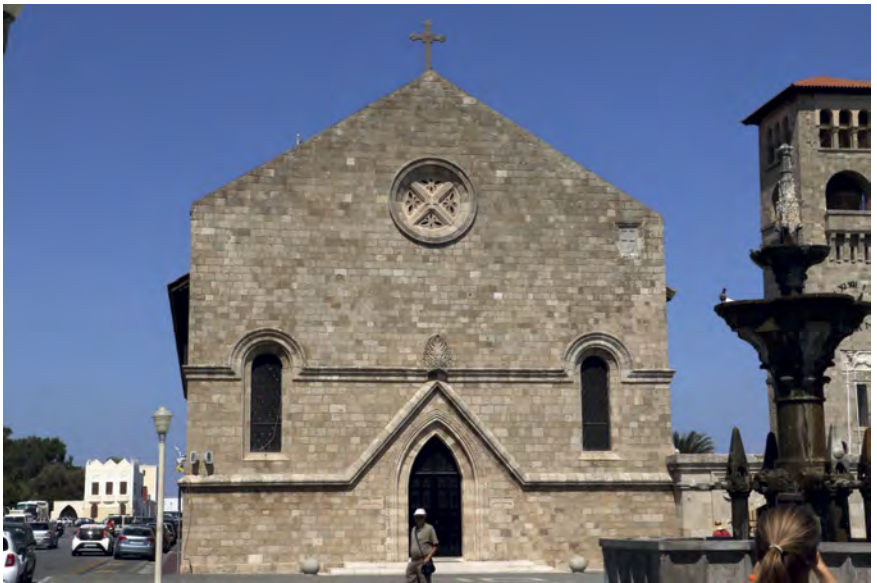
FIGURE 16B The church of the Annunciation, 1924/1925–1929, Mandraki port. View from the west
