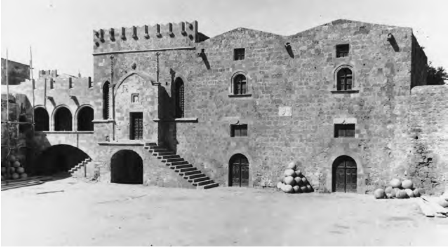
FIGURE 47B The earlier hospital, first half of the 14th century, Rhodes. East facade after the restoration
