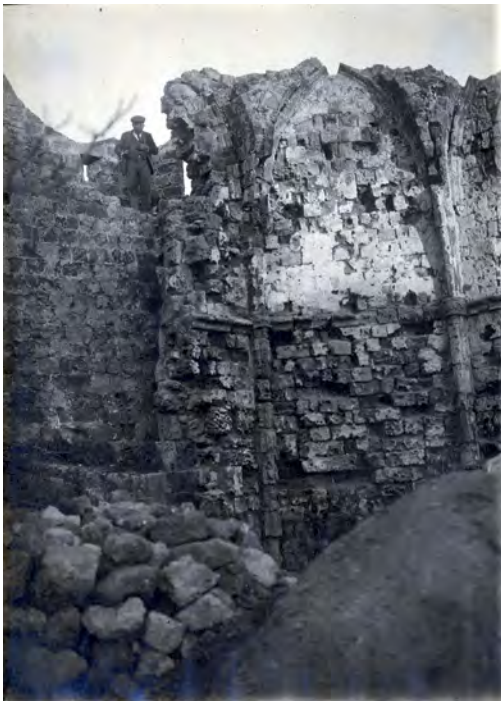
FIGURE 61 Remains of the Gothic apse in contact with the mid-15th-century walls, church formerly identified with Our Lady of Victory, Rhodes
