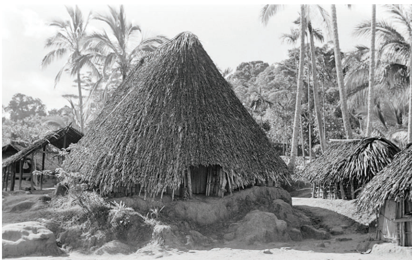
Figure 10. The clan men's house at the Rait hamlet of Bi'ip, 1968. It shows the conspicuous size of the structure and its traditional shape, which is less noticeable in recently constructed men's houses.
