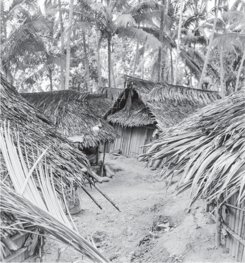
Figure 3. A hamlet with women's individual family houses in the foreground. The thatching of the houses is made from sago-palm leaves, their walls from the large midribs of the leaves.
