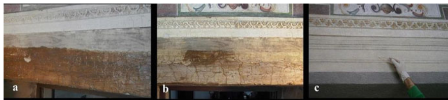
Fig. 11.1 Aged-casein layer covering the architrave over the door at Casina Farnese, Rome. (a) before cleaning, (b) after bio-cleaning with a micro-pack containing UI3 strain, (c) after the pictorial retouching (photo from Mazzoni et al. 2014)
