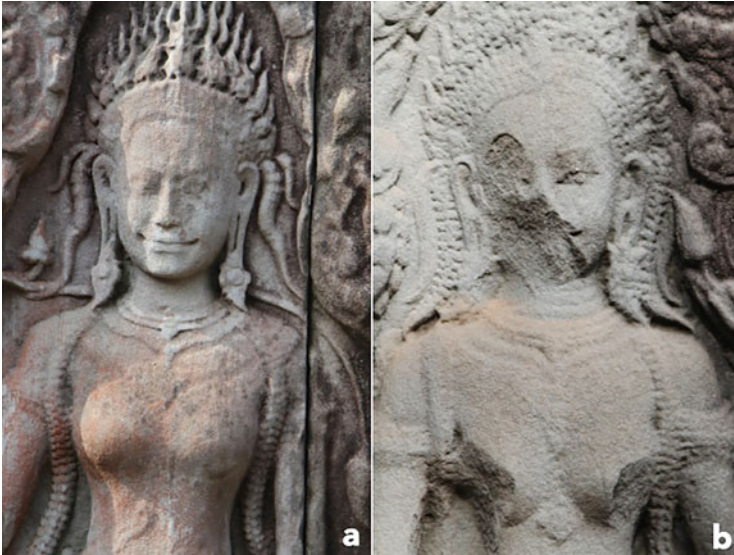
Fig. 2.3 Photographs of Devatas carved on sandstone columns showing differences in conditions and destructions with more red pigment deposition ( a ) and more severe damage ( b ) at Bayon temple of Angkor Thom
