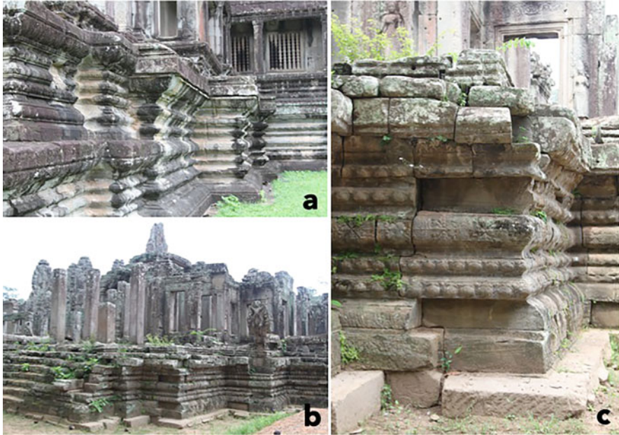
Fig. 2.2 Photographs of the sandstone foundation and current conditions at Angkor Wat (a) and Bayon temple of Angkor Thom from a distance (b) and a close up (c)
