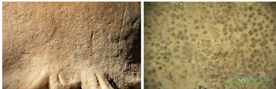
Fig. 1.5 Biopitting on a stone statue, Uffizi Gallery (Firenze, Italy). Close-up of a detail of the surface (right). The circular micro-holes were likely produced by endolithic lichens that grew when the statue was located outdoors. The fruiting bodies were present inside the holes. After the lichens died, they left just the empty holes
