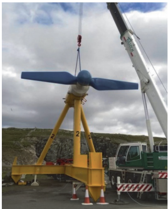
Figure 2. Nova M100 tidal turbine (Source: ©Nova Innovation).
