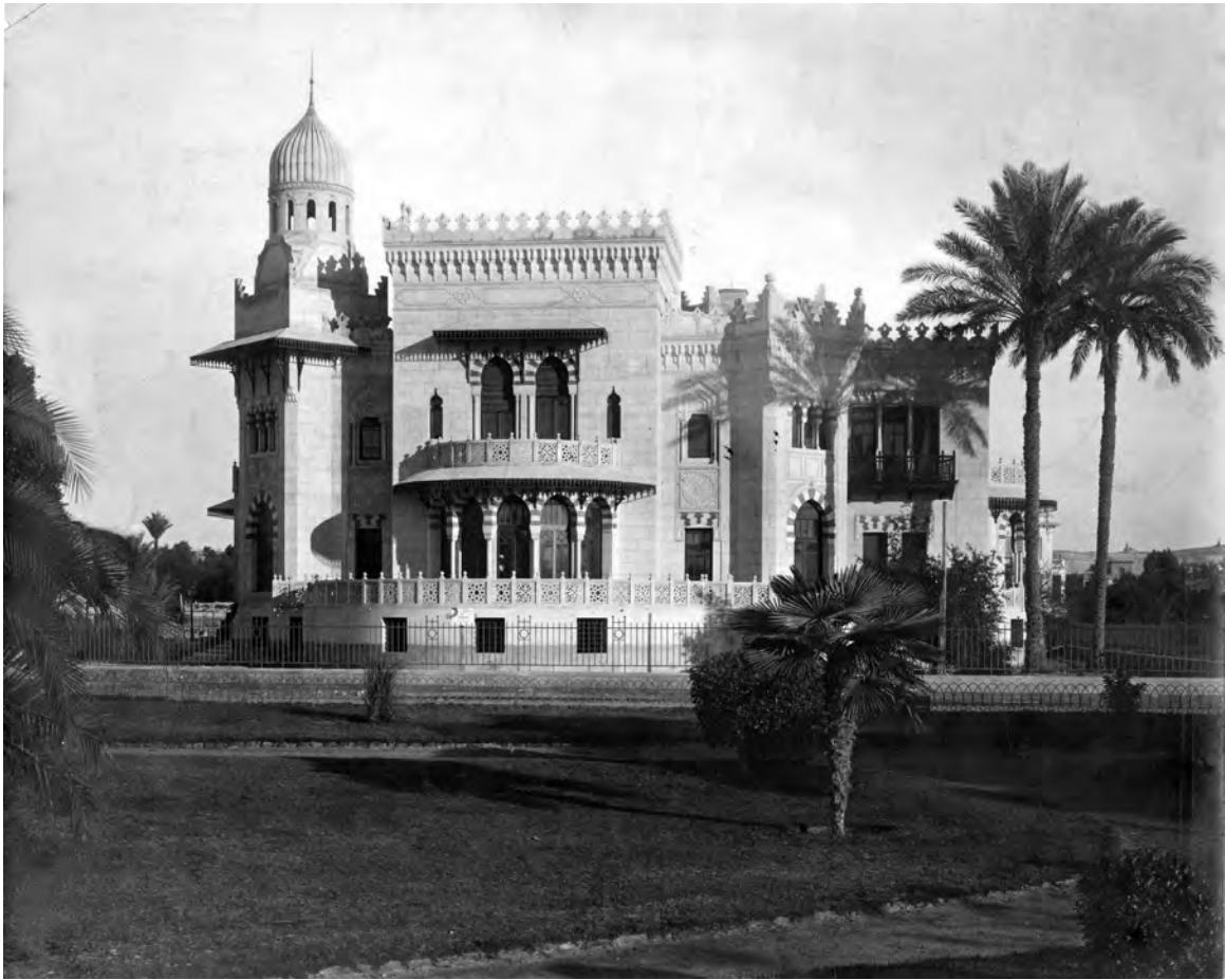
FIGURE 138 Anonymous, Villa Harari , Garden-City (Cairo), undated. The house was built in 1921, architect unknown. Albumen print. 13 × 18 cm PARIS, CENTRE D'ARCHIVES DE L'INSTITUT FRANÇAIS D'ARCHITECTURE, FONDS BÉTONS ARMÉS HENNEBIQUE, 076 IFA, 1-B-160
