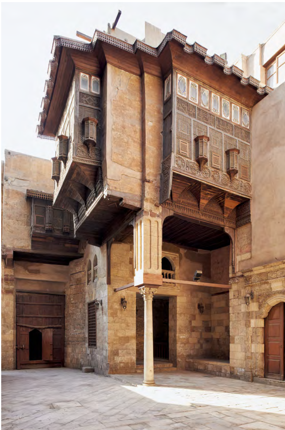
FIGURE 66 An upper qā'a at the house of al-Sadat, resting on a column possibly from a previous construction demolished in the early 1810s PHOTOGRAPH BY MATJAZ KACICNIK, 2016
