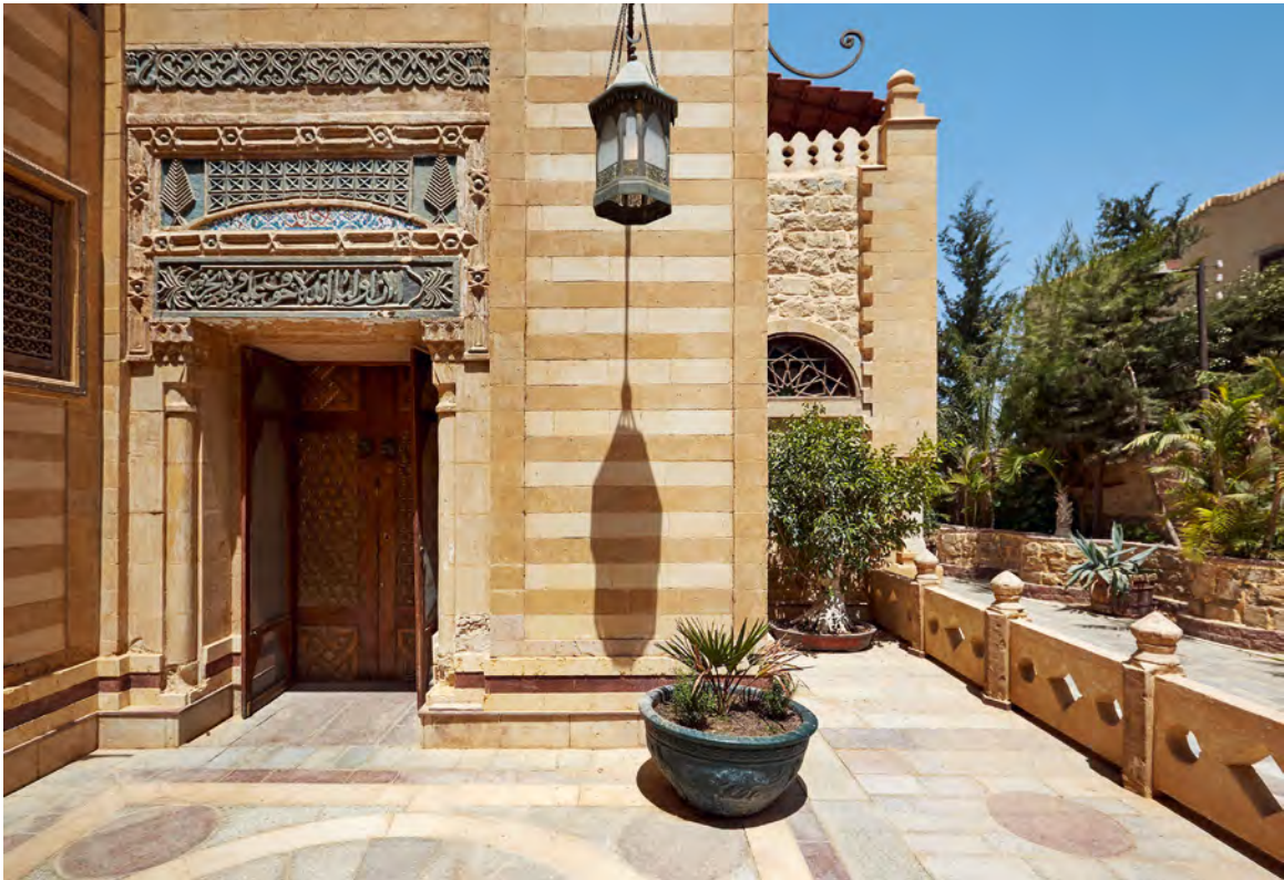
FIGURE 180 Entrance to a house designed by Omar El-Farouk in Fayyum with architectural salvage from the Mosque of Fatima al-Nabawiyya in Cairo PHOTOGRAPH BY HAYSHAM LABIB, 2015
