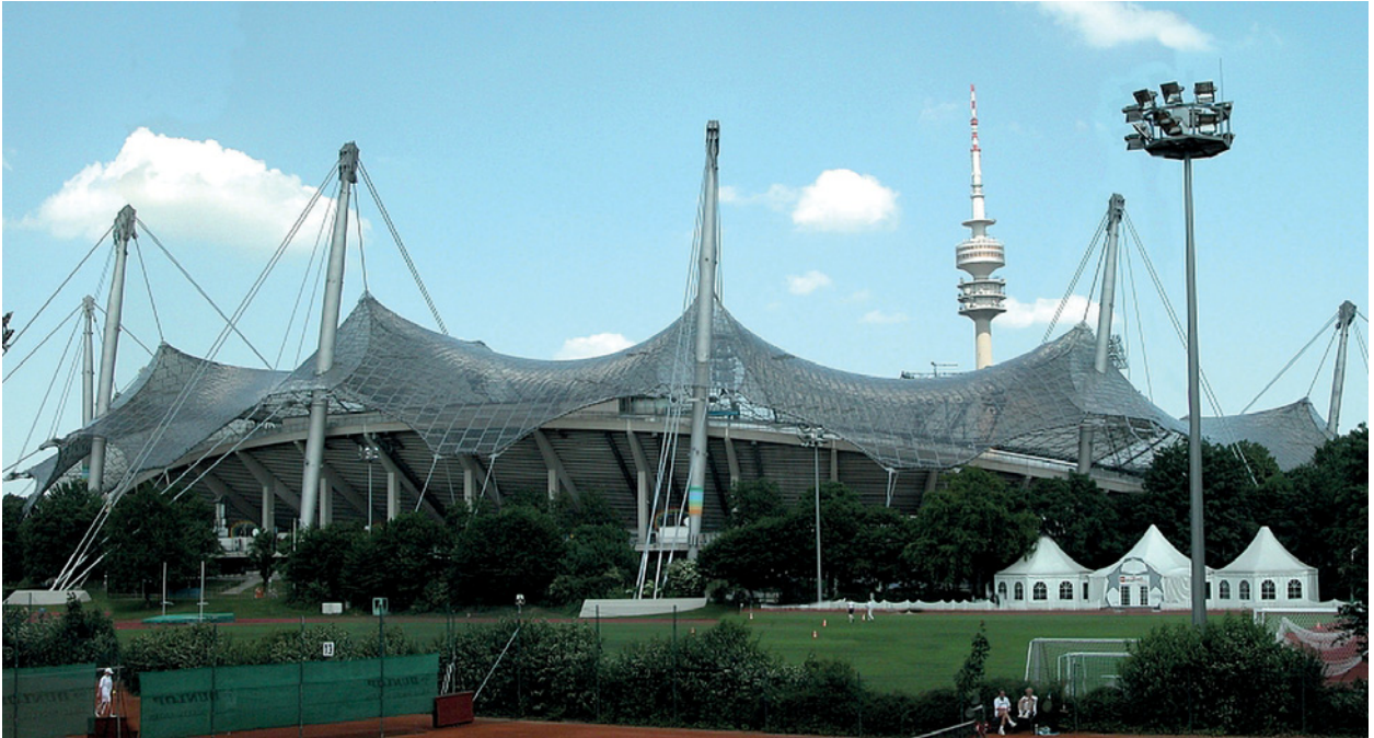
Figure 113: Olympiastadion München, Frei Otto, architect. 1972. Photograph by Fritz Geller-Grimm
