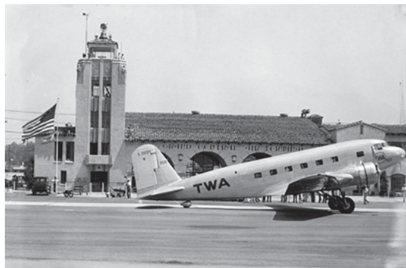
Figure 55: Grand Central Terminal, Glendale, California (1928), photograph courtesy of San Diego Air and Space Museum Archives
