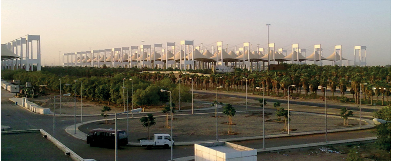
Figure 111: Hajj Terminal at King Abdulaziz International Airport, Jeddah, Saudi Arabia; Photograph by Yousef Madari
