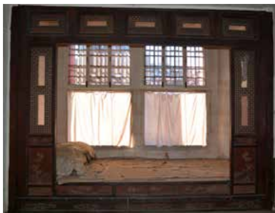
Figure I.1 Decoration and condition of the front bed in Leshou Hall in 2018
