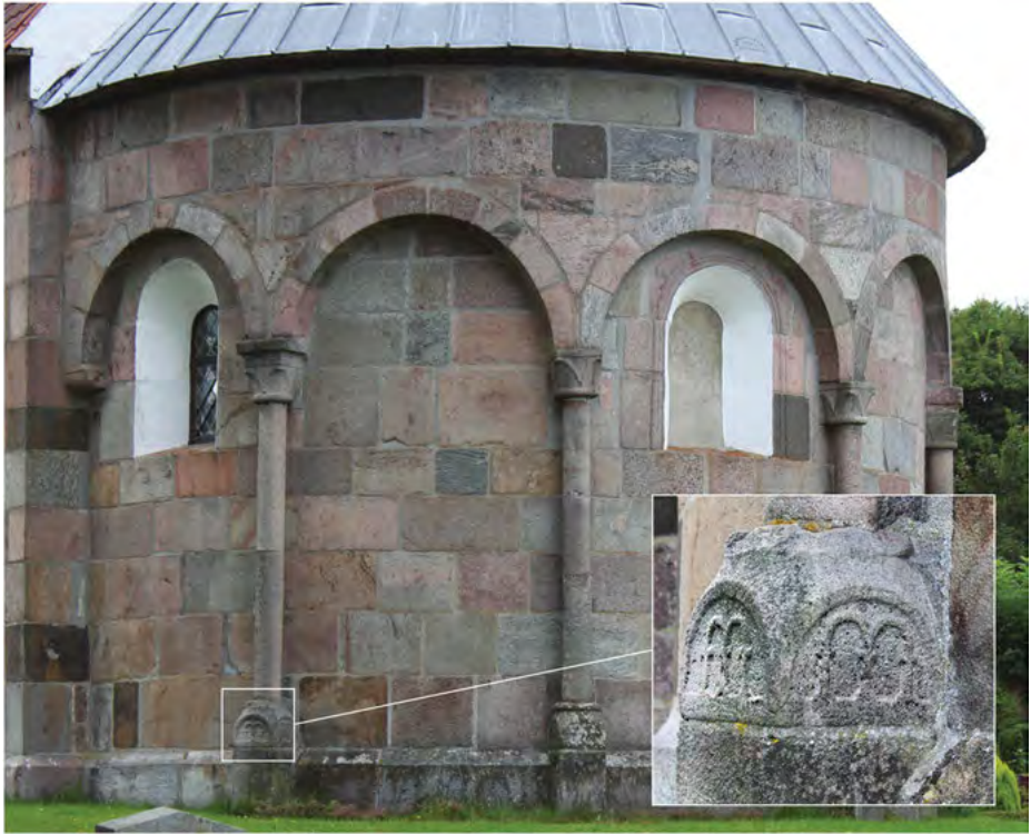
Fig. 15.6: Grønabæk Church, Central Jutland. a. Blind arcades, apse, exterior; b. Detail of column base from the blind arcade of the apse.
