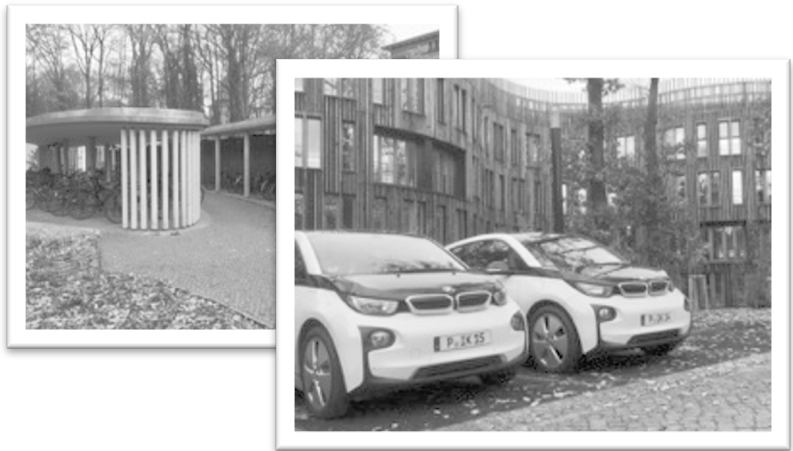
Figure 11: The front of A56 with the parking area for bikes (left) and electric cars (right). Source: Own photo
