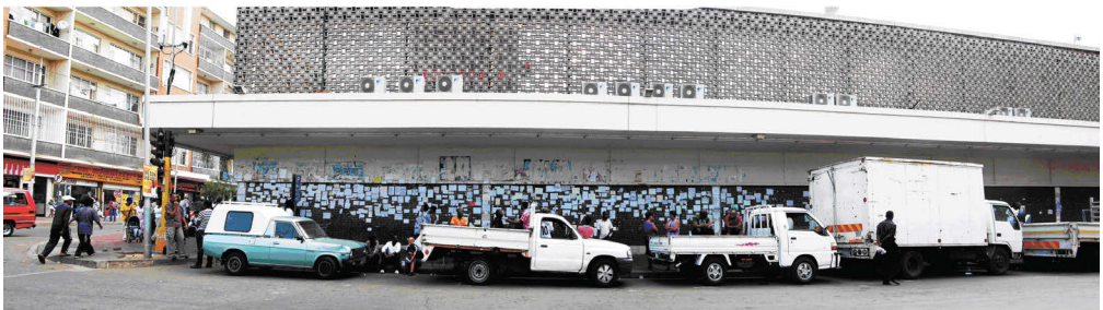
FIGURE 18.2: The rooms and spaces economy at the Shoprite wall
