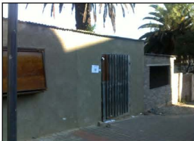
Ugly boundary wall with openings for businesses. Has the property been rezoned for business? Probably not.
