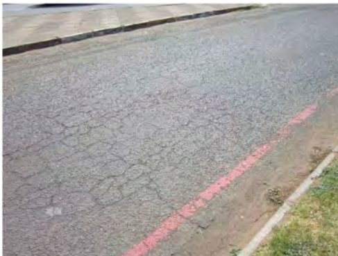
Figure 15. McGregor Street prior to rehabilitation.
