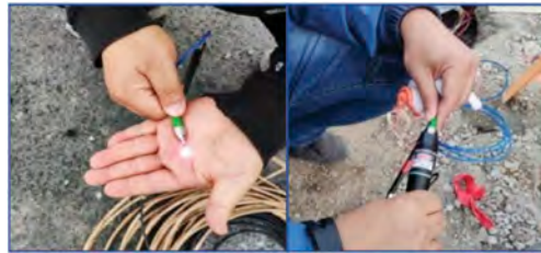
Figure 4. The inspection of the optical fibre sensors.
