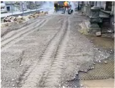
Figure 4. Installation of geogrid.
