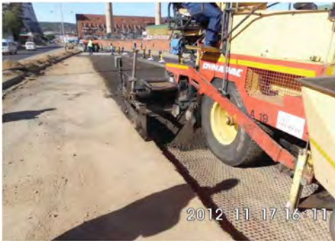
Figure 13. Installation of BSM with paver.
