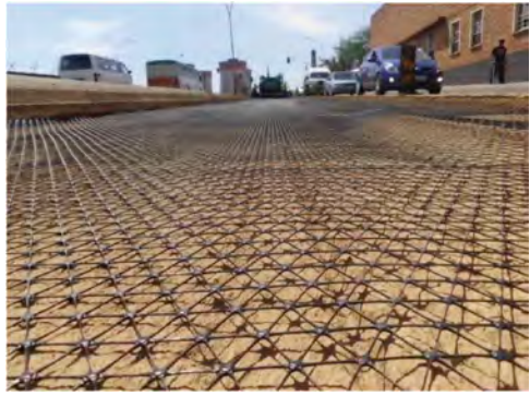
Figure 12. Installation of stabilisation geogrid.
