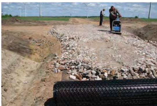
Figure 5. RCA layer stabilised with hexagonal geogrid at Kretinga Wind Farm.
