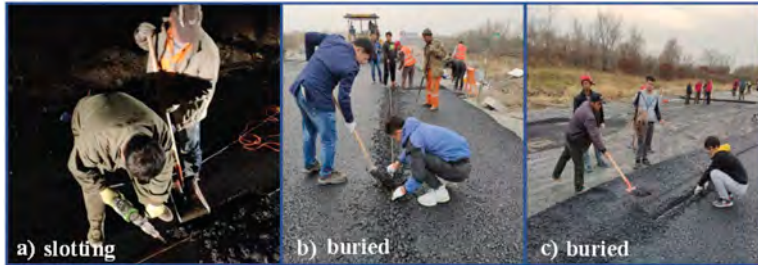
Figure 3. The embedded process of optical fibre sensors in asphalt mixture layer.
