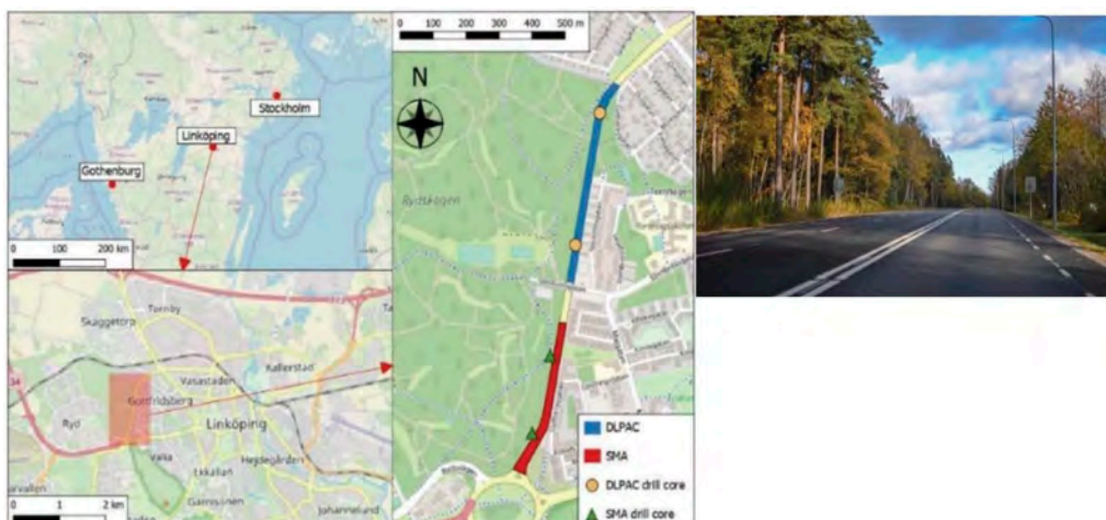
Figure 4. Left: Location of the double layered porous asphalt section in Linköping, Sweden. Adapted from Lundberg et al. (2020). Right: photo of Industriegatan in the northern driving direction at the double layered porous asphalt.
