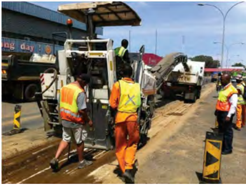
Figure 11. Milling existing asphalt.
