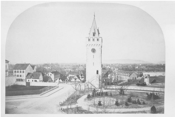
Figure 6: Basel, St Alban's gate with newly laid-out park, around 1875
