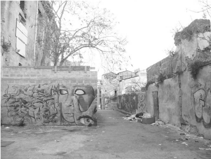
Figure 1: Death, destruction, decay. Albergheria quarter in Palermo (Photo: G. Vinken 2019)
