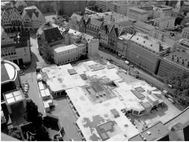
Figure 3: Cleared to build a “historic” town center. Demolition of the “Technisches Rathaus” (Photo: Sarah Bonnert, 2011)
