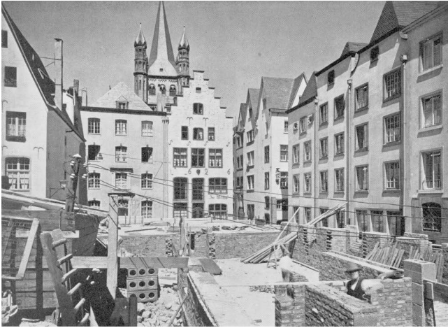
Figure 9: Cologne, rehabilitation works at the Eisenmarkt square, 1938
