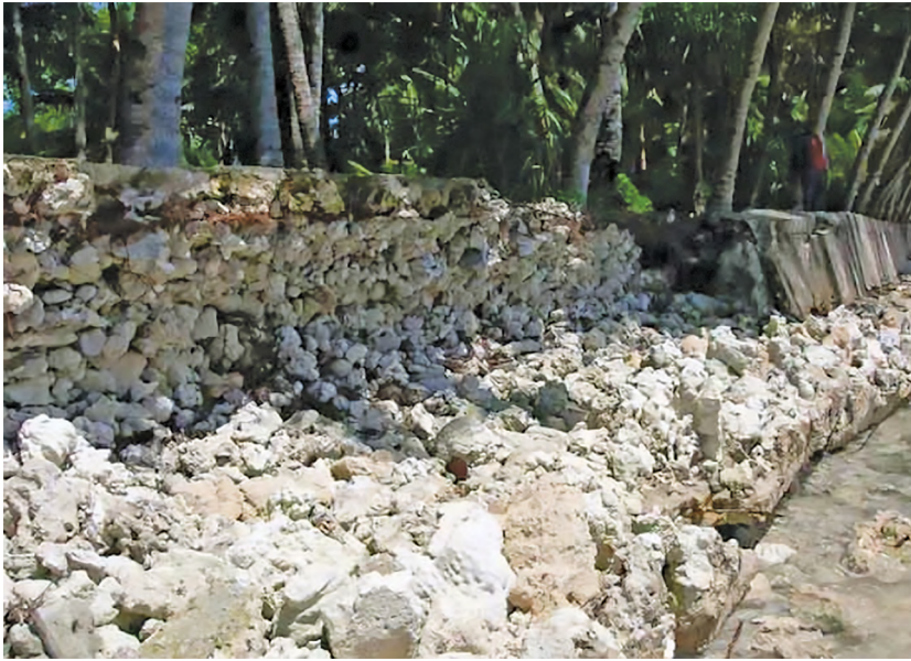
Figure 16: Old-style seawall constructed in the 1970s on the island of Lukunor.
