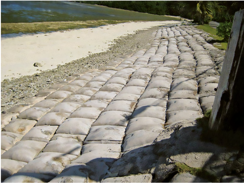
Figure 17: New seawall design in Kosrae to prevent beach erosion.
