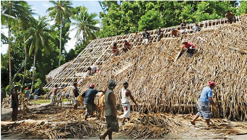
Figure 18: People of Rewow village, in 2014, on Lekinioch work to replace pandanus sheets on foeng, the ainang faal of Sopunpi, demonstrative of the principle of allis fengen .
