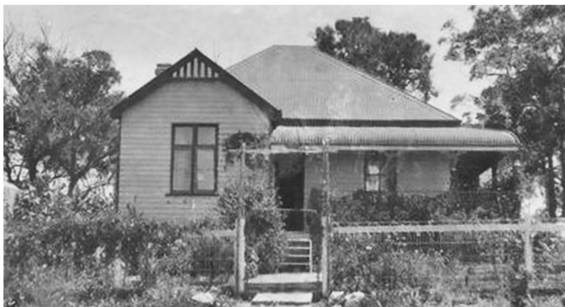
Figure 7.1: The manager’s house at Roseby Park Aboriginal Station.
