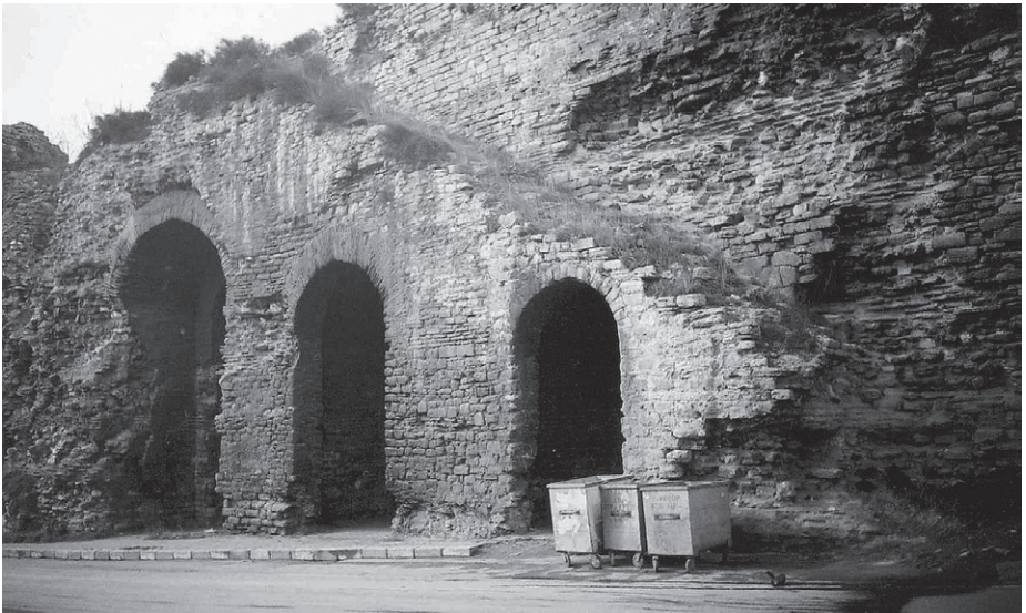
Abb. 94 Landmauer, Sulukulekapı, Wehrgangtreppe
