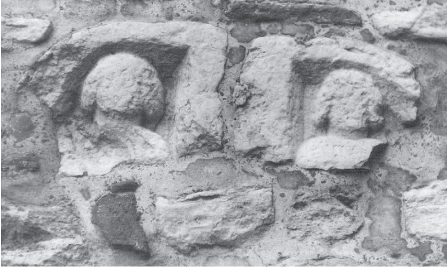
Abb. 209 Marmara-Seemauer, Turm 17, Akrotere (1999)
