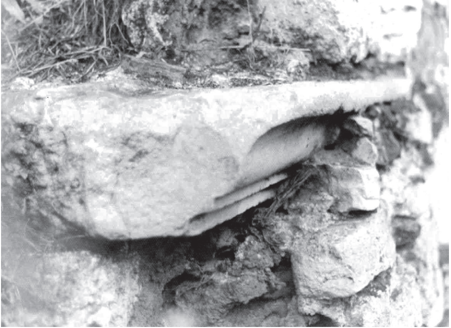
Abb. 186 Landmauer, Kurtine 18/19, Türsturz-Fragment
