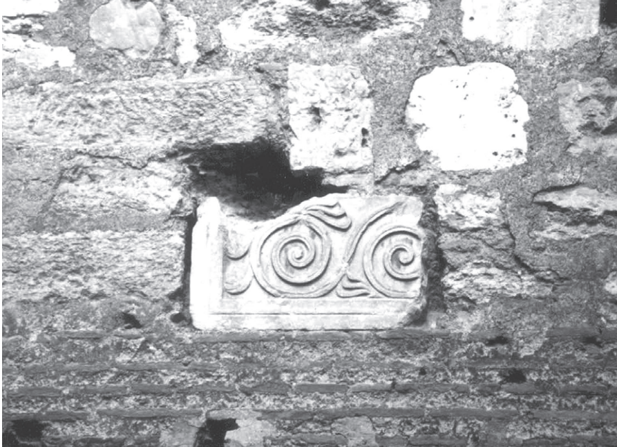
Abb. 192 Komnenen-Mauer, Kurtine 8/9, Platte
