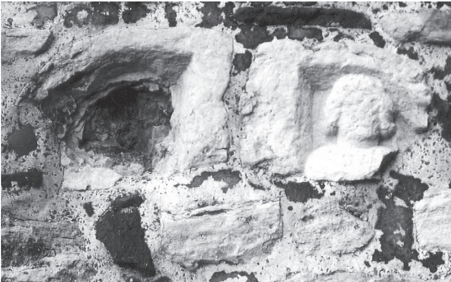
Abb. 210 Marmara-Seemauer, Turm 17, Akrotere (2000)
