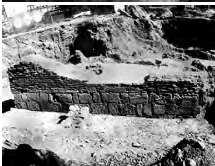
Fig. 5.2. Southern early Byzantine wall with a pentagonal tower – view from the north
