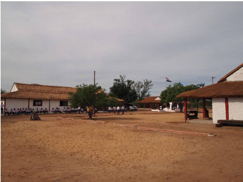
Figure 5.8b A partly restored Fortín Isla Po'í in June 2013 (Source: author).
