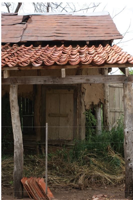
Figure 6.7 Mennonite house with sheet-metal roof made of flattened oil canisters from the war (Source: author).
