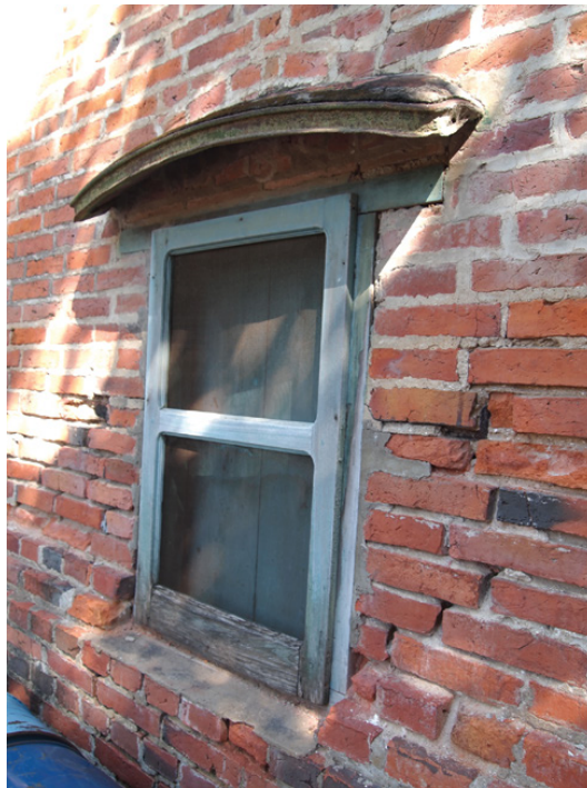
Figure 5.2 Bent railway track serving as decoration above a window (Source: author).
