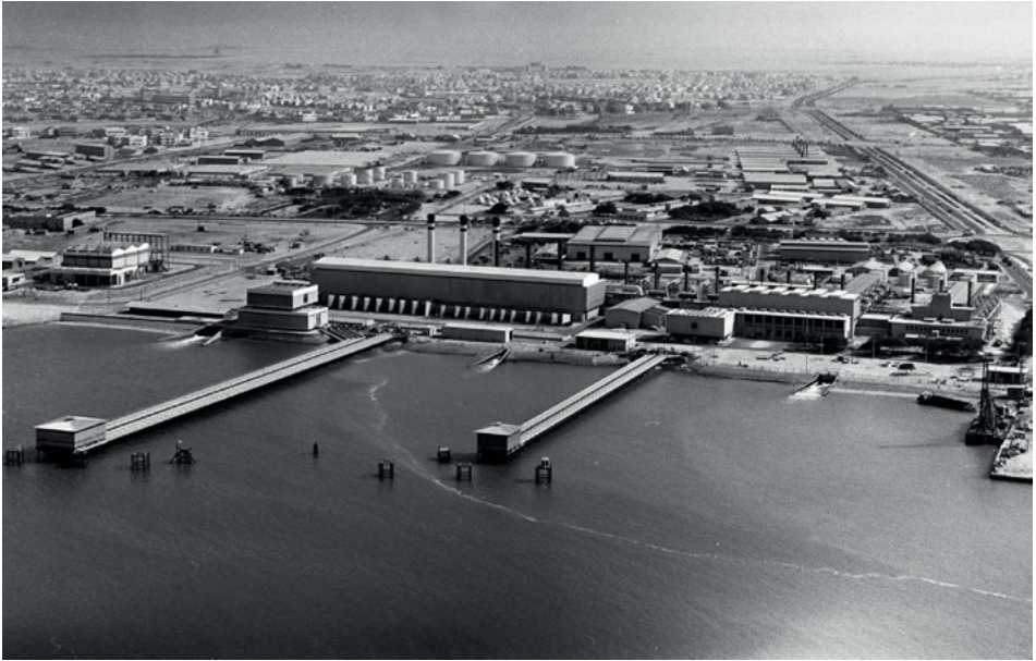
5.12 Black-and-white oblique photograph of the power and desalination plant in Shuwaikh, Kuwait City. Undated, photographer unknown.
