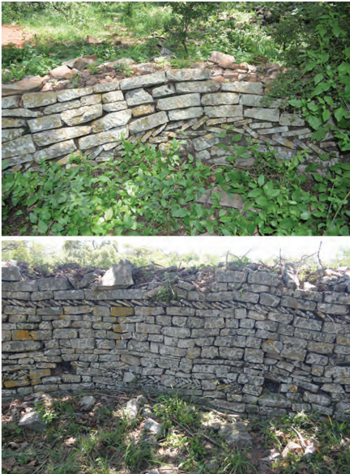
FIGURE 4.10 (A) Interior and less visible decoration at Nsalansala, central Zimbabwe; (B) Interior and less visible decoration at Shangagwe, central Zimbabwe
