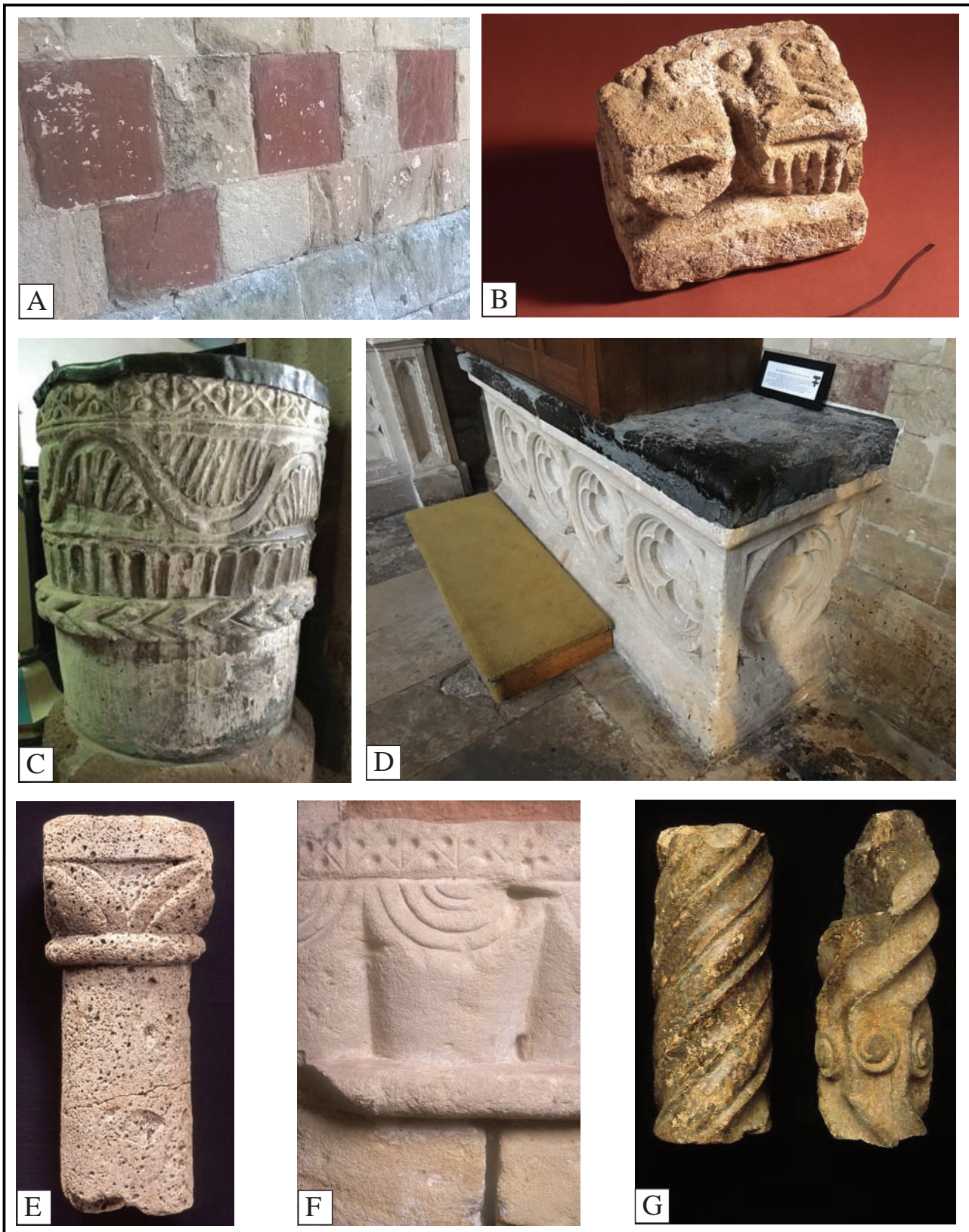
Fig 7.23 The market in building stone in 12th-century Exeter. (A) Triassic Red Rock Sandstone at the cathedral. (B) Salcombe stone at St James Priory. (C) Beer stone at Mary Steps church. (D) Grey Lias at the cathedral (tomb slab attributed to John the Chanter). (E) Volcanic Trap, St James Priory; (F) Triassic sandstone, St Nicholas Priory. (G) Purbeck marble, St Nicholas Priory (photos: B, E–G: David Garner; A and D: John Allan; C: © Alex Woodcock)
