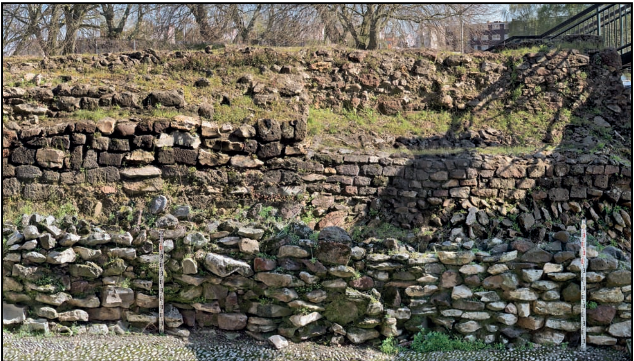
Fig. 6.9 Roman rear facework and footings of the inside face of the City Wall in South Street/Western Way (photo by Gary Young; © Exeter City Council)
