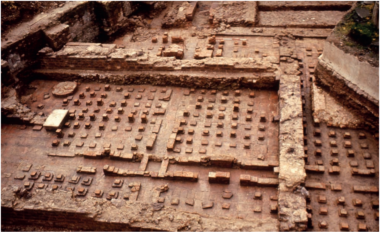
Fig. 5.9 The caldarium of the fortress baths looking south-west towards one of the two furnaces which served it. Note channels dividing the hypocaust into four segments so as to distribute the heat more evenly. The wall crossing the room from left to right represents the front of the later basilica; part of the tepidarium to the right (© RAMM)
