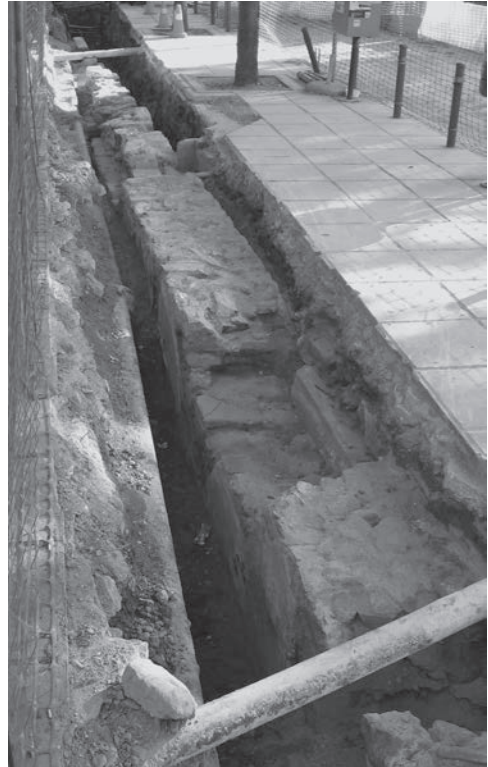
Fig. 10.5: Excavations during the installation of Thessaloniki's new water pipe (N. Bakirtzis).
