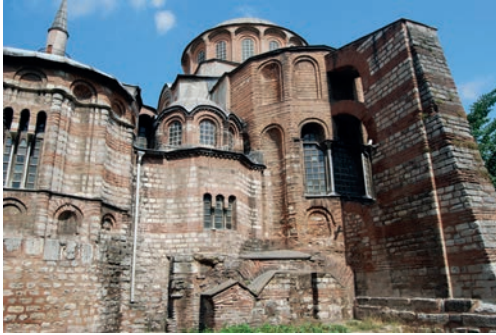
Fig. 3.9: Istanbul. Kariye Camii, view from east, showing multiple phases of construction (author).
