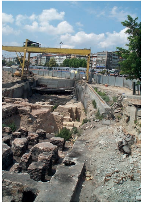
Fig. 3.3: Istanbul. Excavation for subway, near Aksaray, revealing multiple strata of architecture (author).
