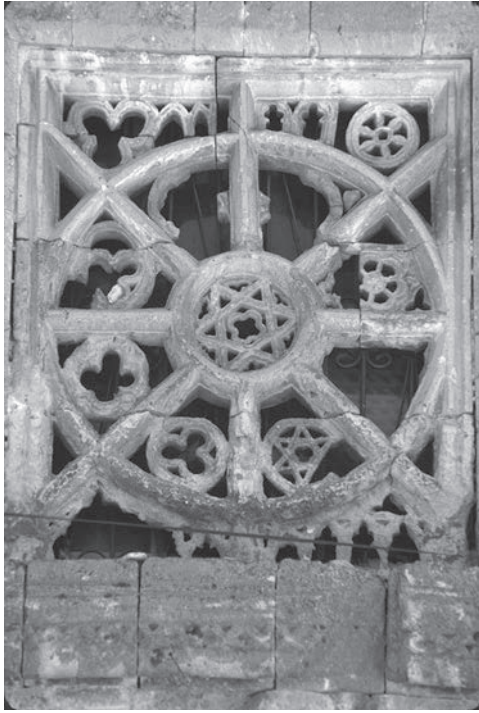
Fig. 4.5: Sungur Ağa Mosque, window detail, north portal (author).
