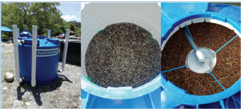
Figure 4.27. INNOQUA lumbrifilter created with locally available materials in Cuenca. Images courtesy of Andrés Alvarado, showing (left to right): an external view; gravel layer; splash plate distribution system.
