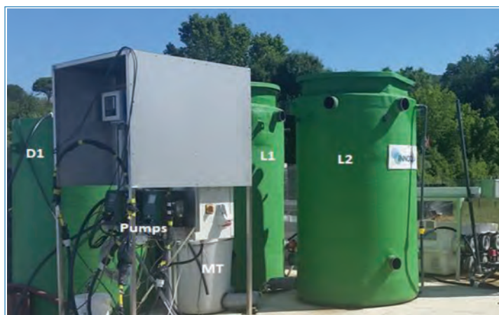
Figure 5.12. INNOQUA integrated system at the UDG pilot-site (Quart WWT, Girona, Spain). The system consisted of two 5 PE lumbrifilters (L1 and L2), a mixing tank (MT) and a 10 PE Daphniafilter (D1).
