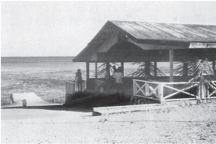
Figure 5. Small wharf, facing entrance through reef ( avanui ), and fare kako , Tauhunu, where welcoming ceremonies are conducted for important visitors to Manihiki.
