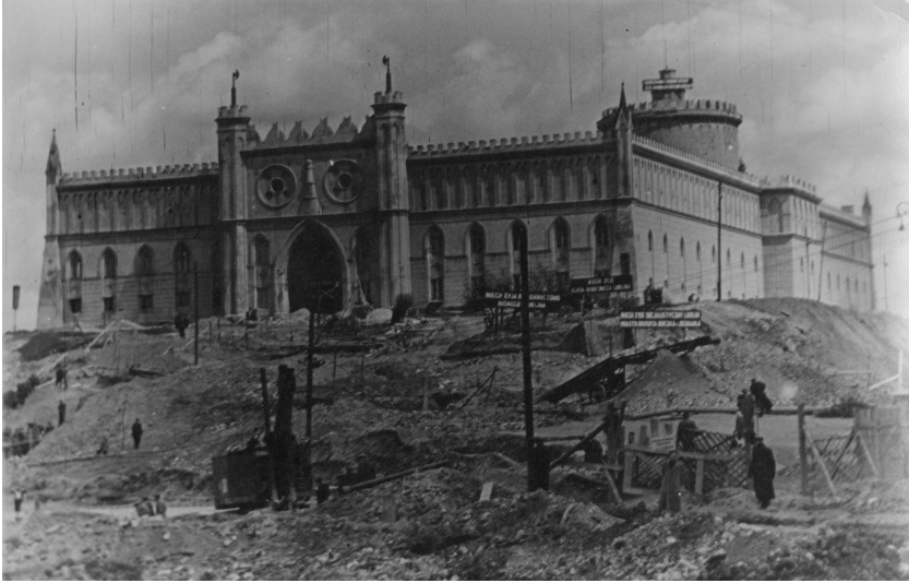
Figure 7.3 Construction of the People's Meeting Square (former Castle square).
