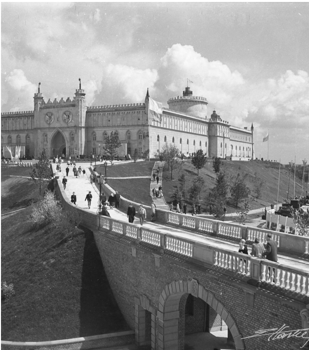
Figure 7.5 Lublin Castle Viaduct.
