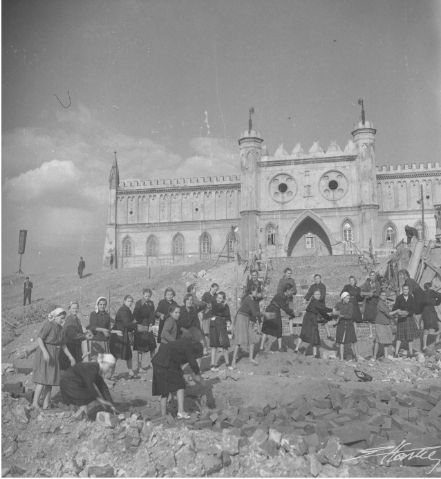
Figure 7.2 Construction of the People's Meeting Square (former Castle Square), 1954.
