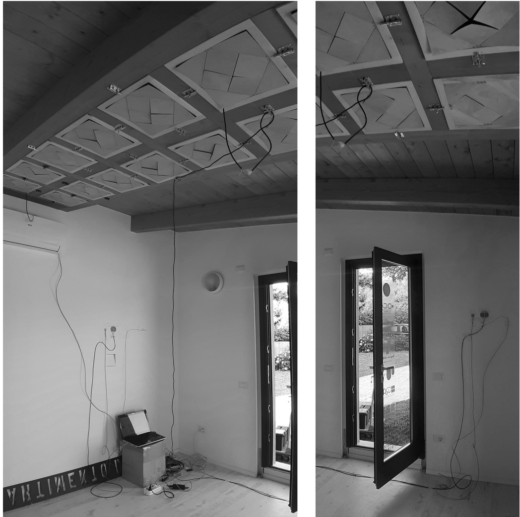
Fig. 2. Thermocouples, fluxmeters, temperature and humidity probes and anemometers inside the test room.
