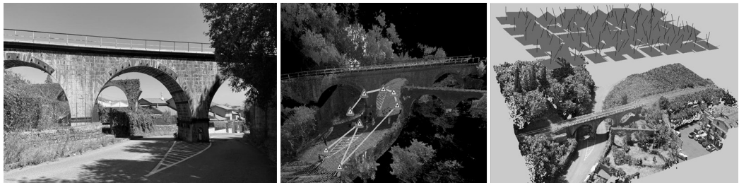
Fig. 1. The result of the survey campaign for a three-arch bridge in the municipality of Mascali (CT). The instruments used are: a NIKON D5300 (photogrammetry), Leica BLK360 (TLS), DJI MAVIC 2 PRO (UAV photogrammetry).
