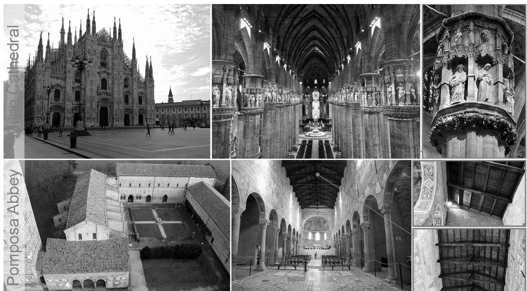
Fig. 1. External and internal photos of the Milan Cathedral and Pomposa Abbey, with details of the monumental capitals of the Cathedral and the wooden roofs of the Abbey (authors' images).
