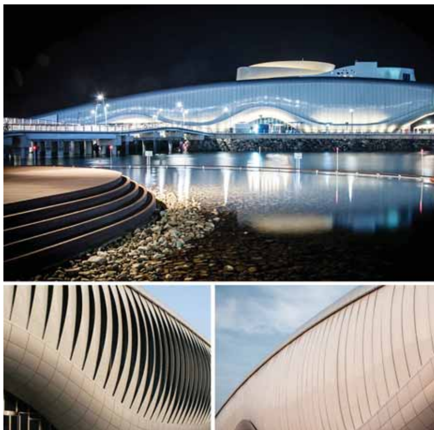
Fig. 4.4 - Soma Studio. Thematic Pavilion for Yeosu Expo 2012 (©Soma). The design's concept for the 140 meters long and 3 to 13 meters height dynamic façade originated from biology and is an example of a central level system. The 108 kinetic lamellas controlled internal light conditions and created organic external animated patterns. Servomotors reduced the distance between the two bearings to originate the movement, resulting in a side rotation of the lamellas.
