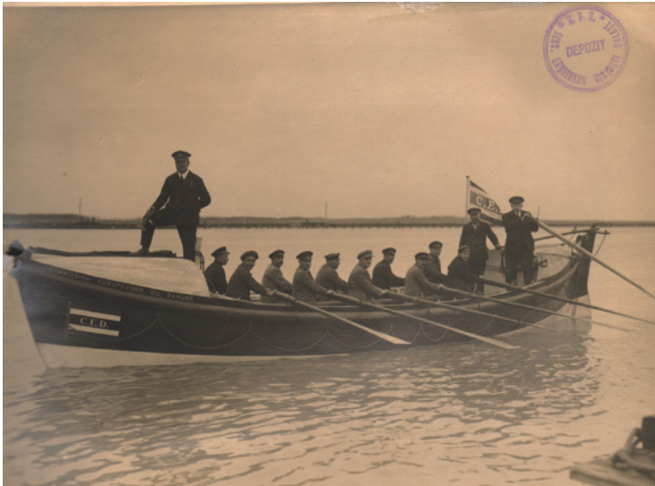
FIGURES 13-14 The lighthouse of Sulina and the Rescue Service (1930) SOURCE: THE NATIONAL ARCHIVES OF ROMANIA, GALAȚI BRANCH
